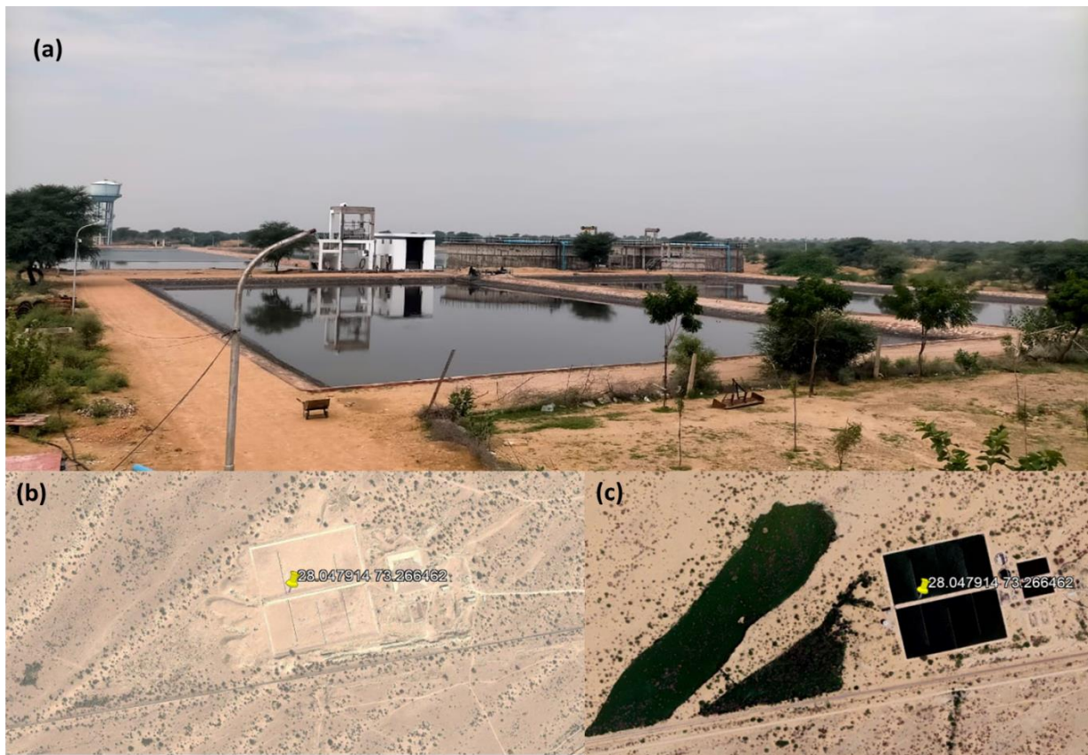
Figure 10.2B: Existing STP located in Sarah Nathaniya, Bikaner ( 28.047914^{\circ} N, 73.266462^{\circ} E) being upgraded to SBR Technology (Capacity of plant is 12.0 MLD) (a) Field photograph (b) Satellite imagery in 2015 (c) Satellite imagery in 2021
