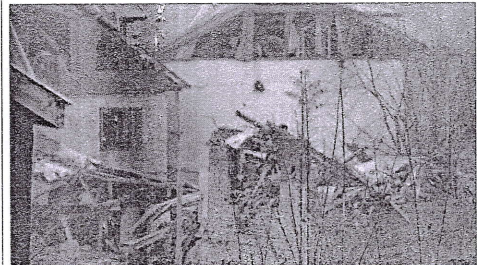
A damaged building inside the Nowgam police station premises on the outskirts of Srinagar. R1
