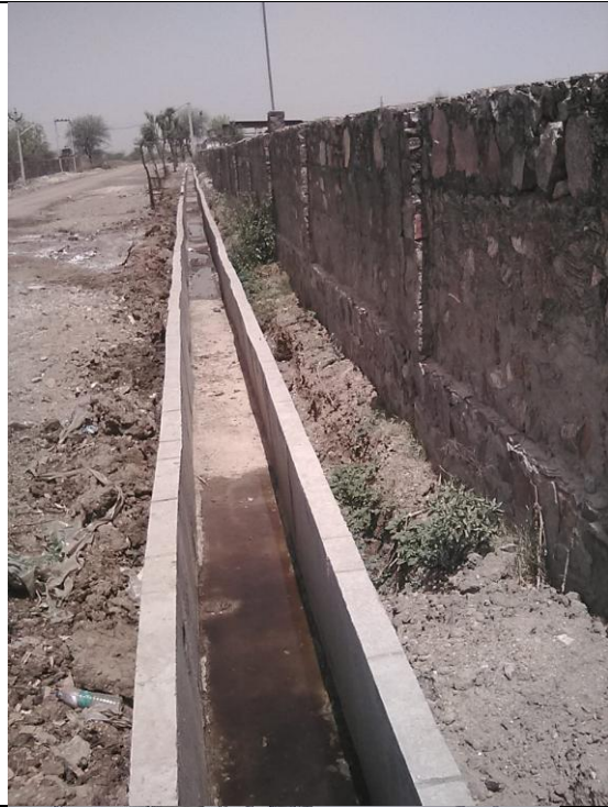
Development works (RCC Drain & Approaches) IA Malpura
