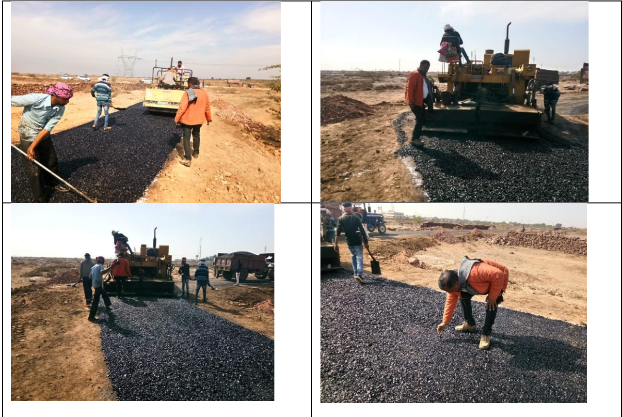
Construction of Road at IA Masalpur (Running work)
