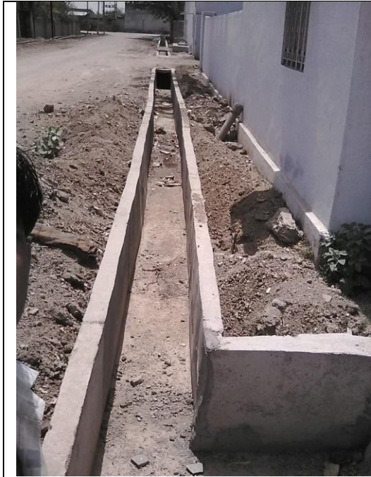
Development works (RCC Drain & Approaches) IA Malpura
