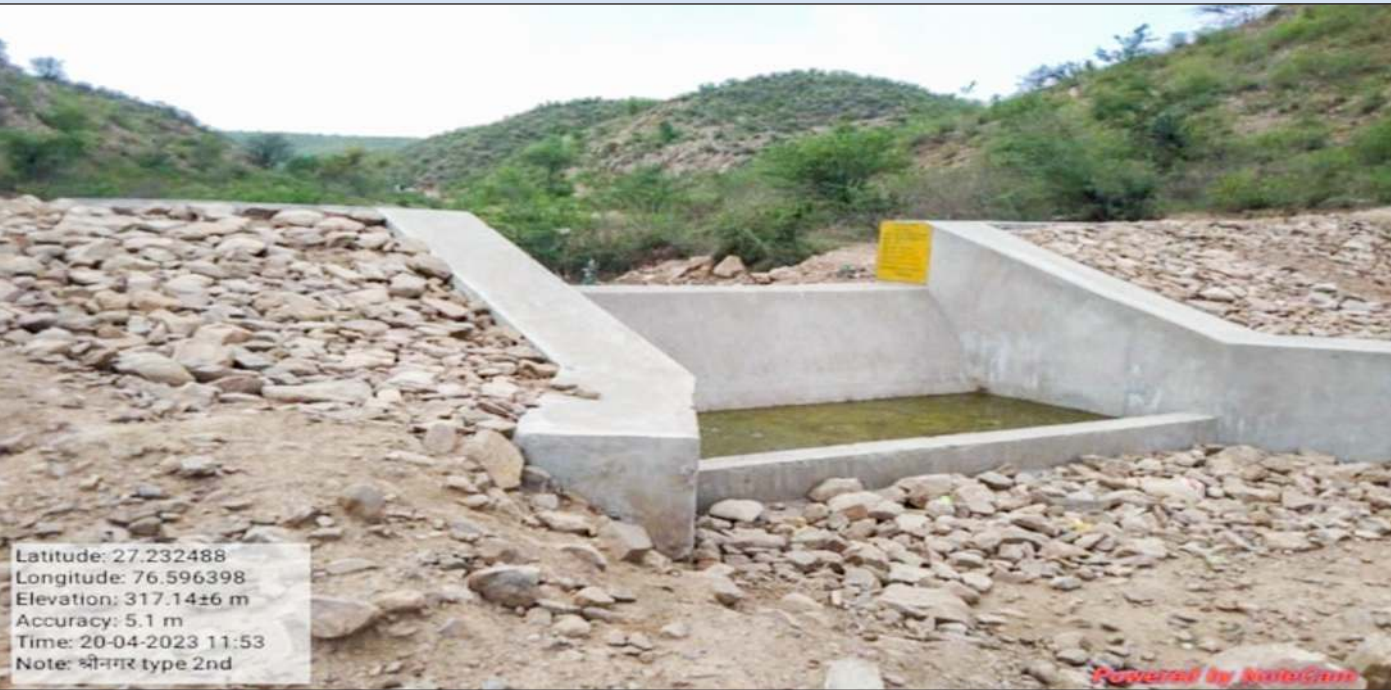
Construction of Anicut Type II at Shri Nagar in Alwar division (Year 2022-23)
