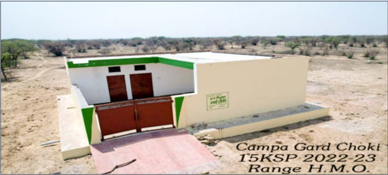
Forest Guard Chowki and Office-cum-Range Officers' Residence constructed at Tonk Division in the Year 2022-23
