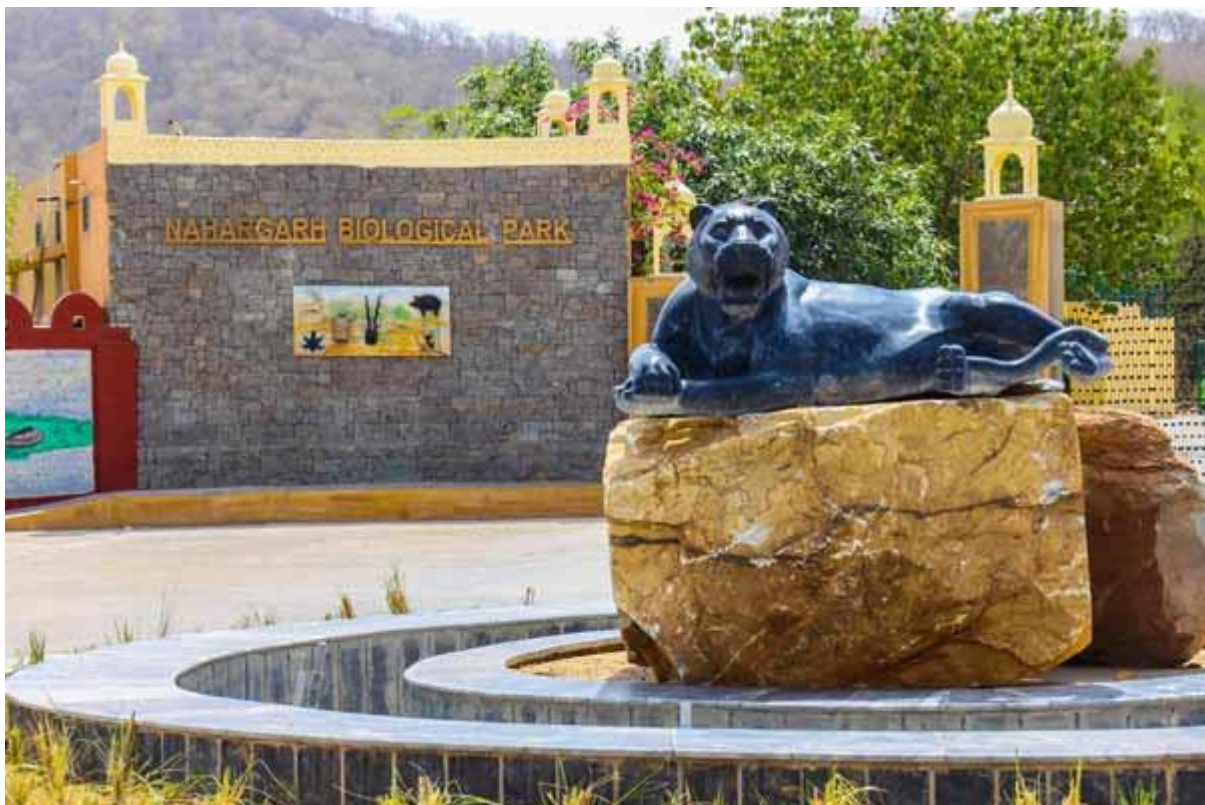
Figure No.: 13.2 Existing Site Photograph of Nahargarh Biological Park
