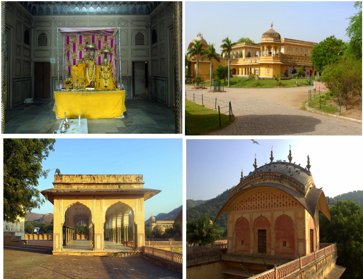
Figure No.: 12.14 Images of the existing structures at Old Govind Ji Temple
