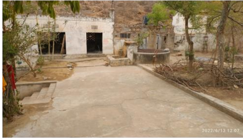
Kitchen and Existing Pathway
