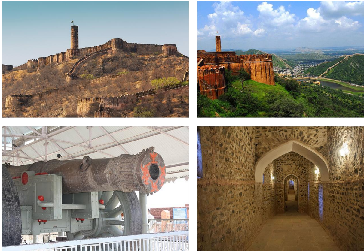
Figure No.: 13.18 Facilities Available in Jaigarh fort
