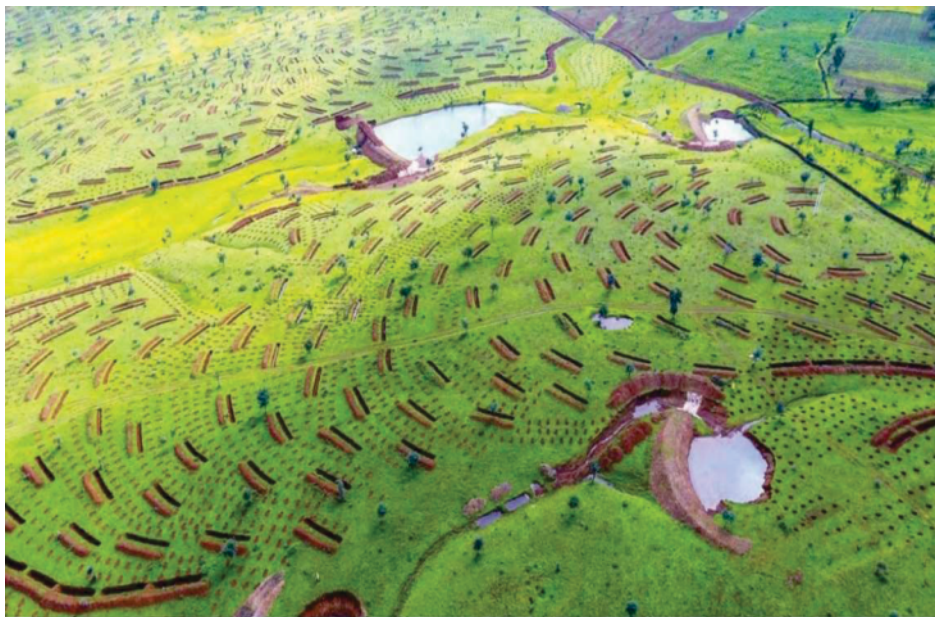
Figure 19 : Images of CCT and SGT works constructed under MJSA-I in the Rajasthan
