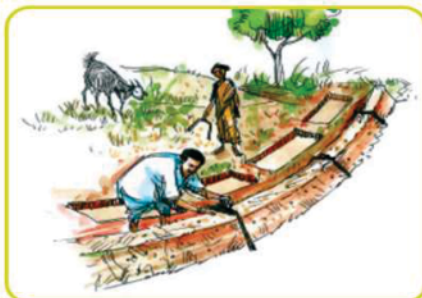
Checking the section of the bund with a template
