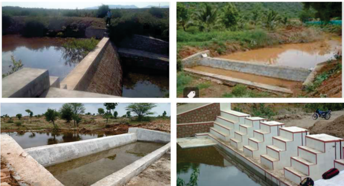
Figure 36 : Images of various masonry check dam
