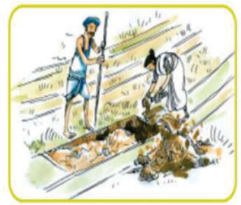
Digging trench and keeping soil on downstream side
