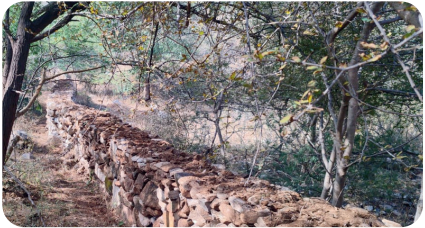
MIGRATORY BIRD COUNT, RESTORATION OF FENCING WALL
