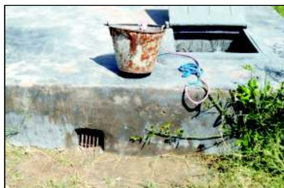
Water Harvesting Tank at Mander Site. (October – 2012)
