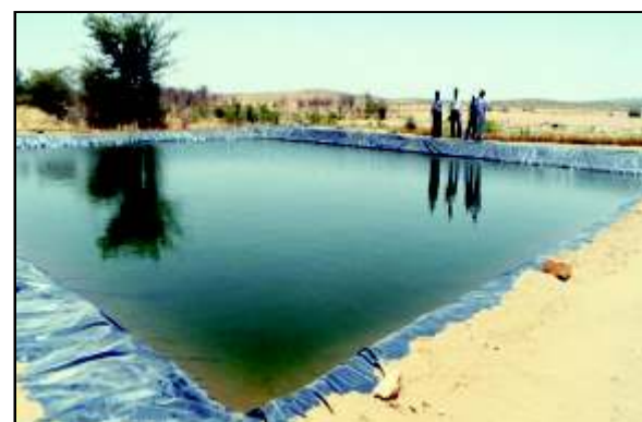
Emergency Reservoir for nurseries at Gadara Sub Branch Canal, Jaisalmer
