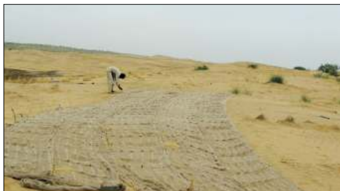
Step – 1 : Laying of the Jute Mesh Mulch
