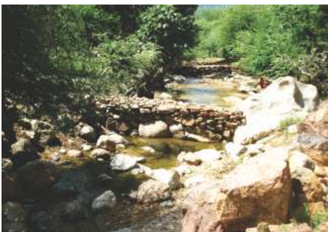
Package : Water Conservation Structure Activity : Gabion Structure DMU : Jalore
