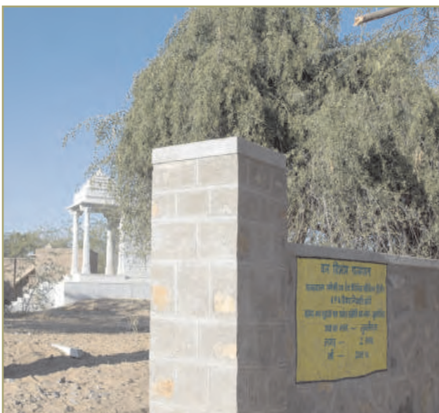
EPA - Construction of boundary wall, Jubliganj, Sirohi
