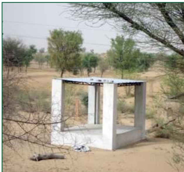
Entry Point Activity - Shed in the Samsan Bhaleri VFPMC, Churu
