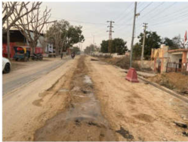
Laying of Pumping Main DI pipe from SwPS Parmana taal to Disposal Point towards Mega Highway, Sardarshahr
