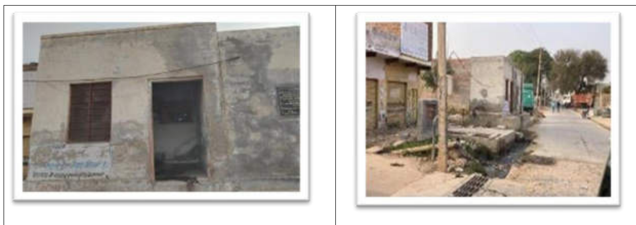
Figure 3: Photographs of the Existing SWPS – 2
