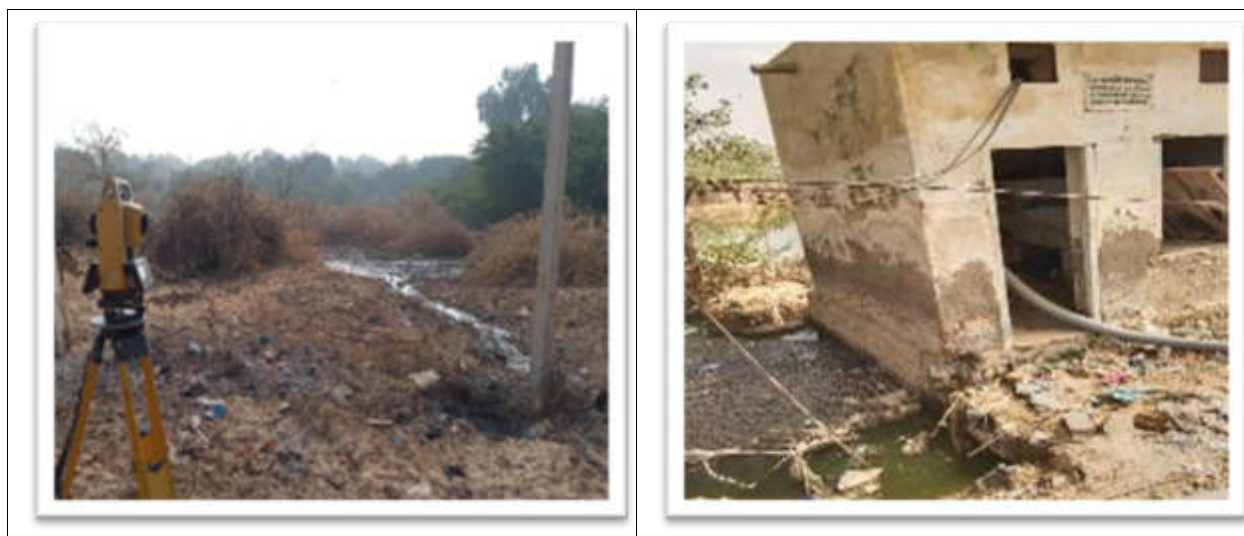
Figure 4: Photograph of the SWPS – 3 Site
