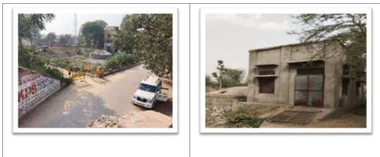
Figure 6: Photograph of the SWPS-5 Near BSNL office
