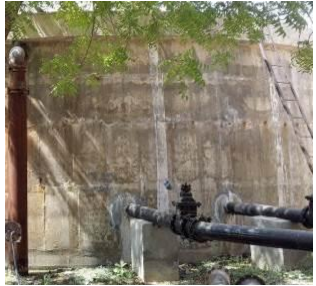
CWR at Samdari headworks
