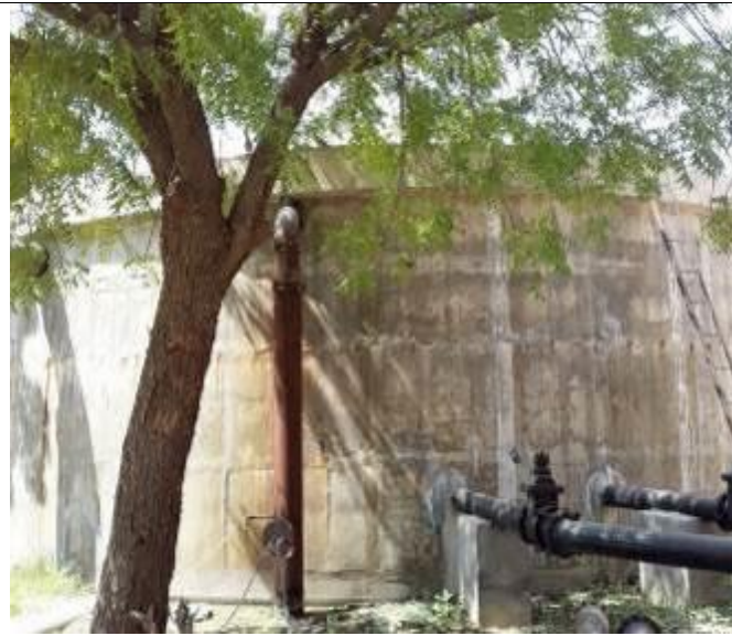
CWR at Samdari headworks
