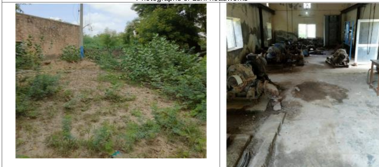
Photographs of Samdari headworks
