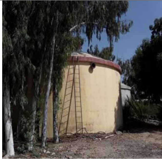
CWR at Luni headworks
