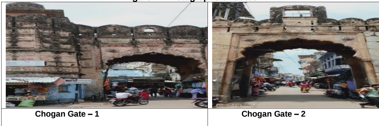
Figure 4: Photographs of Gates
