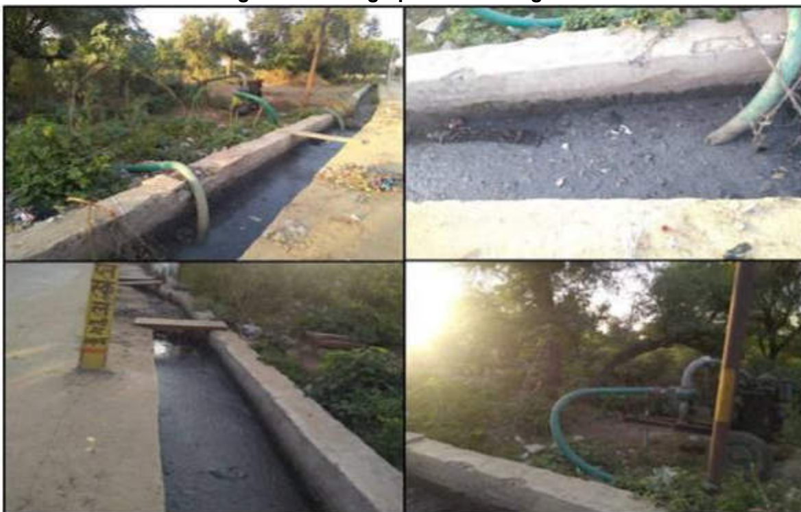
Figure 2: Photographs of Existing Drains
