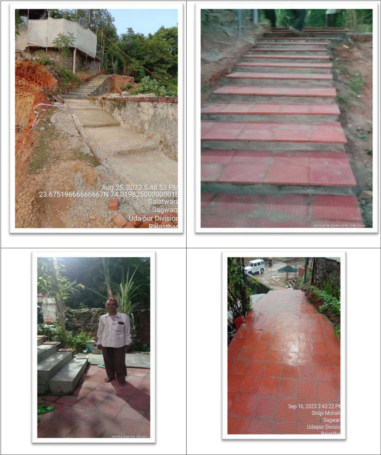
Figure A: Progress of Works of Staircase of temple Sri Ambey Mataji, Sagwara
