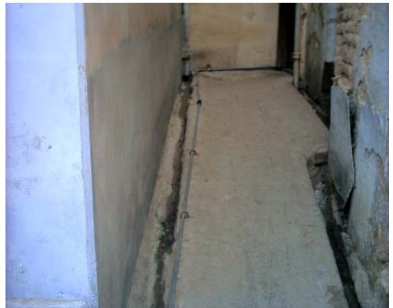
Photo 10: Piped Water Supply in Alwar
