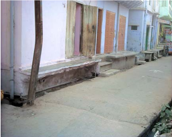
Photo 19: Encroachments into ROW in Alwar
