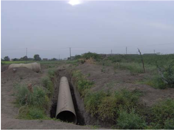
Photo 1: RCC Sewer Pipes
