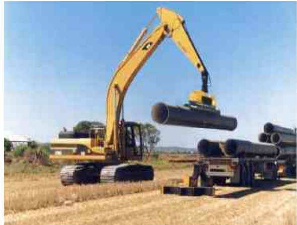
Photo 22: Crane for placing pipes in trench
