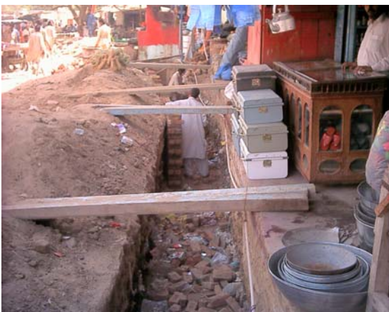
Photo 21: Digging a trench by hand
