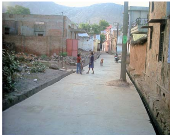
Photo 11: Roadside Concrete drains in Alwar
