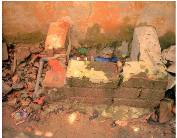
Photo 4: Household water meter
