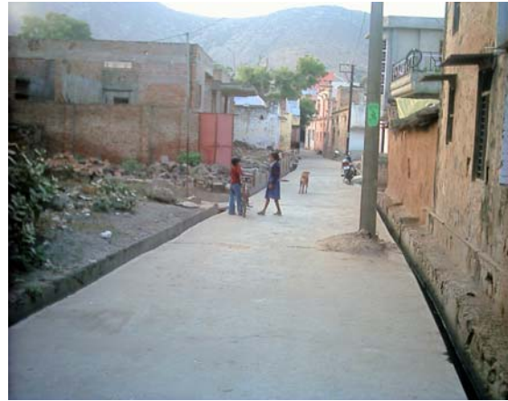
Photo 9a: Roadside drains in Alwar
