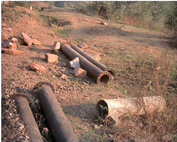
Photo 2: Ductile Iron water pipes
