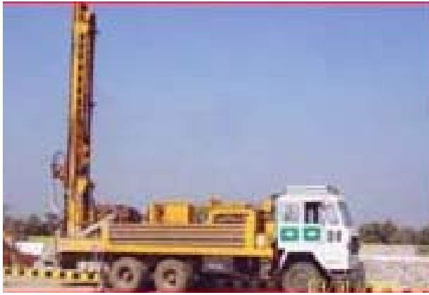
Photo 17: Rig used to drill tubewells
