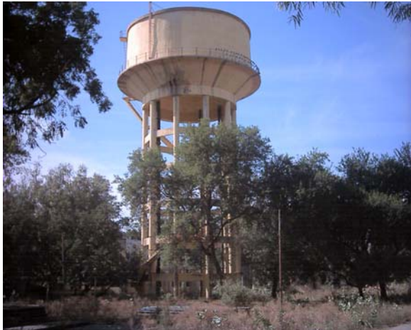
Photo 1: Overhead Reservoir in Alwar
