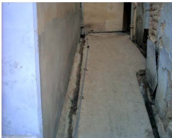
Photo 3: Above ground water supply pipes
