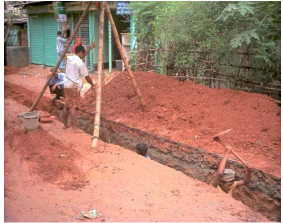
Photo 19: Digging a trench by hand
