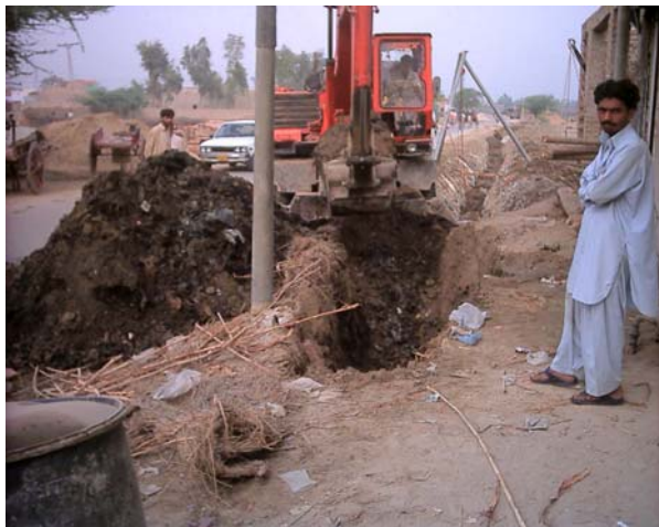
Photo 18: Backhoe digger constructing a trench
