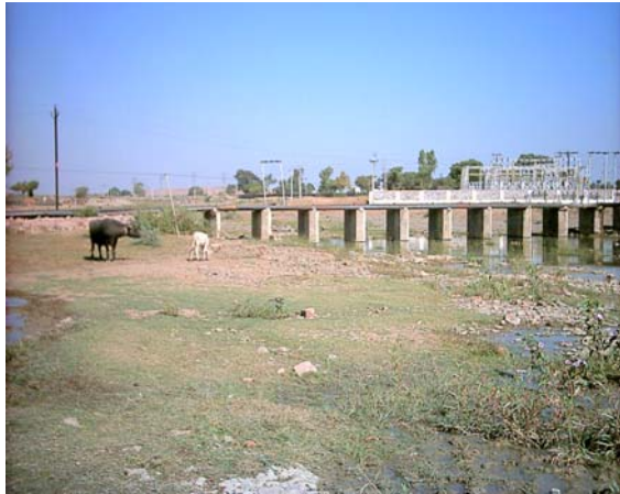
Photo 12: Piped water supply in Jhalrapatan
