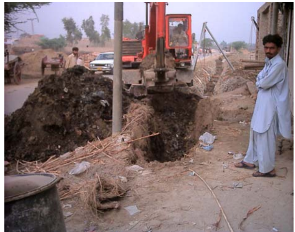
Photo 22: Backhoe digger for trenching
