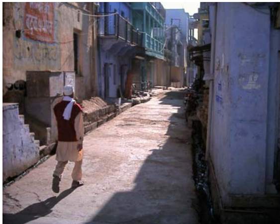
Photo 13: Roadside drains in Jhalawar
