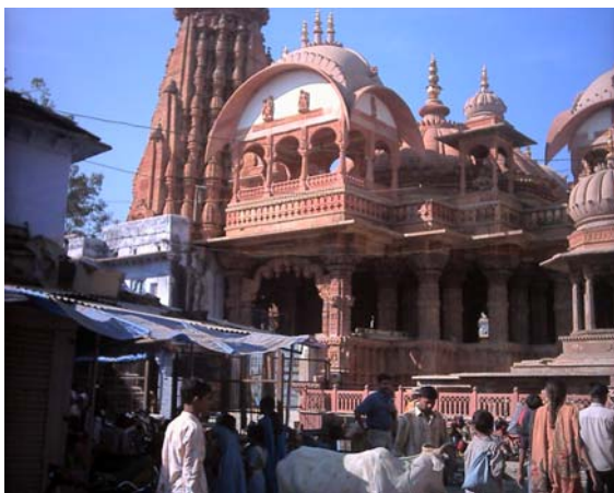
Photo 20: Surya temple, Jhalrapatan
