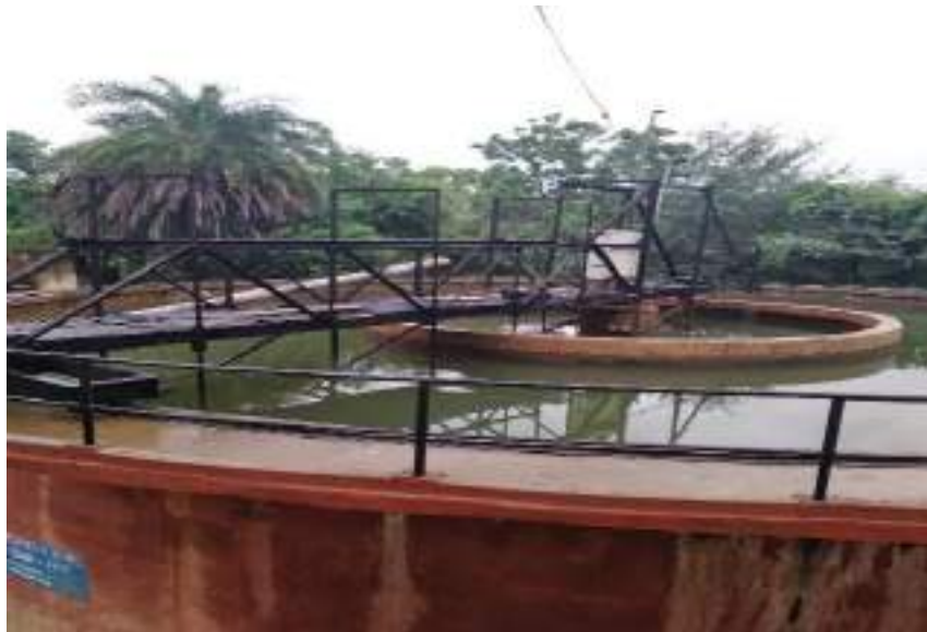
Figure 2 : Udai vilas clarifloculator
