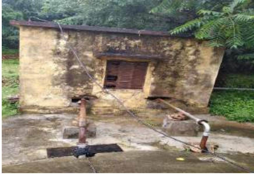
Figure 6 : CWR at Udaivilas (113 KL)
