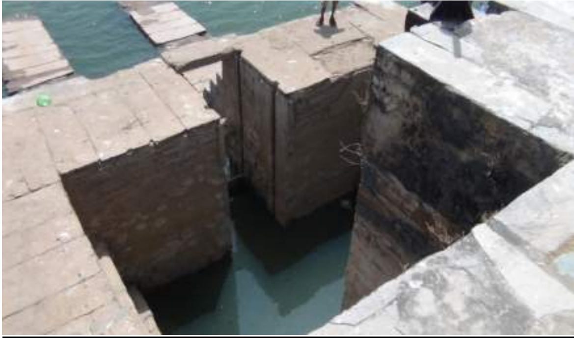
Fig. 11 Intake as Edward Sagar Dam
