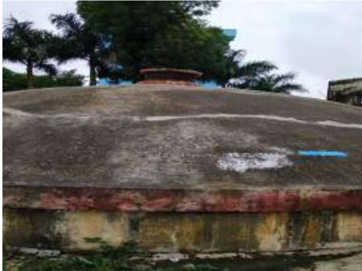
Figure C-9 : CWR at Bori head works (325 KL)
