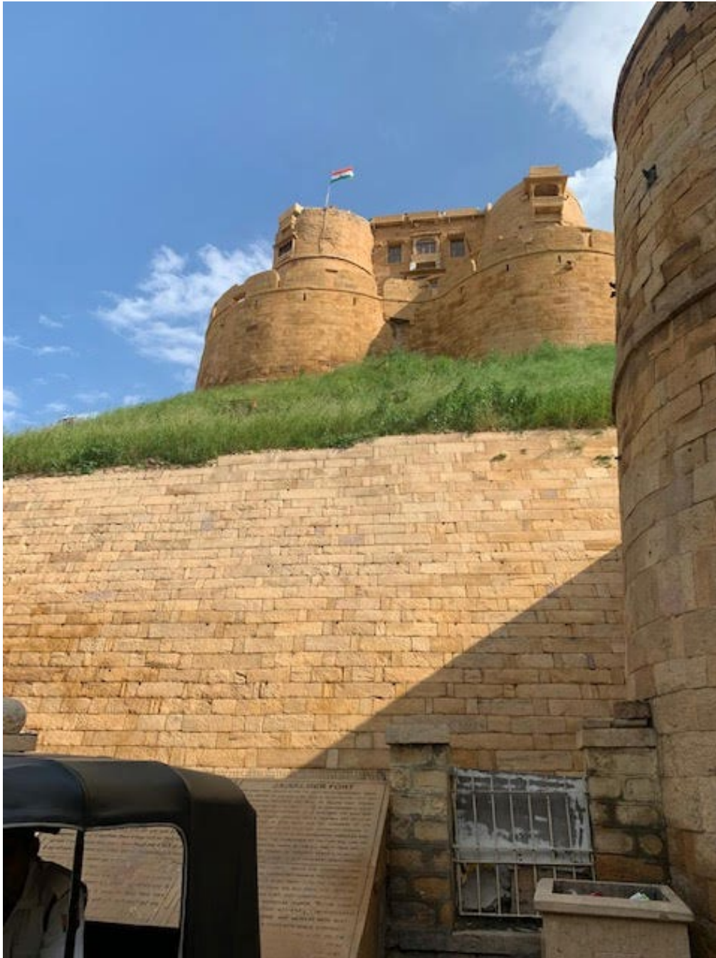
Historic fort wall (multi-level with soft treatment along slope), stone walls, stone pitching in stepped profile with green area to break the monotony of the masonry and allow for drying action
