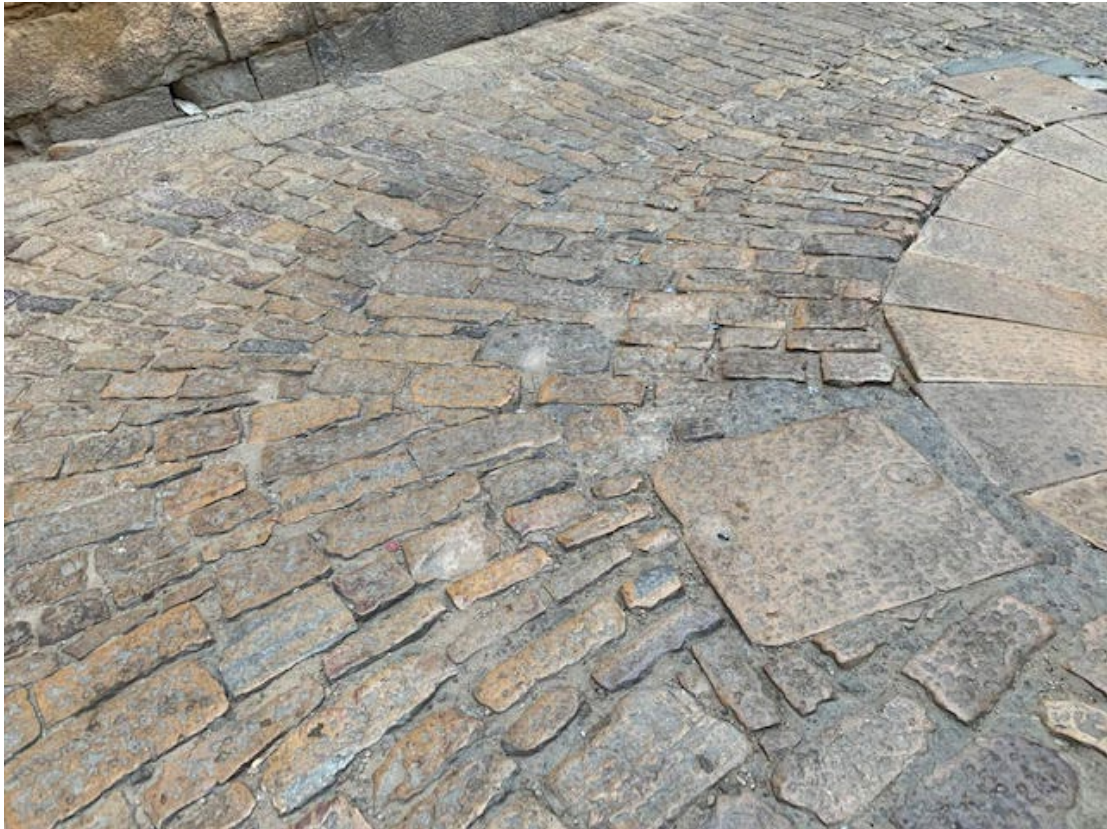
Dry stone paving on the road leading into the Jaislamer fort provides reference for paving materials and construction technique
