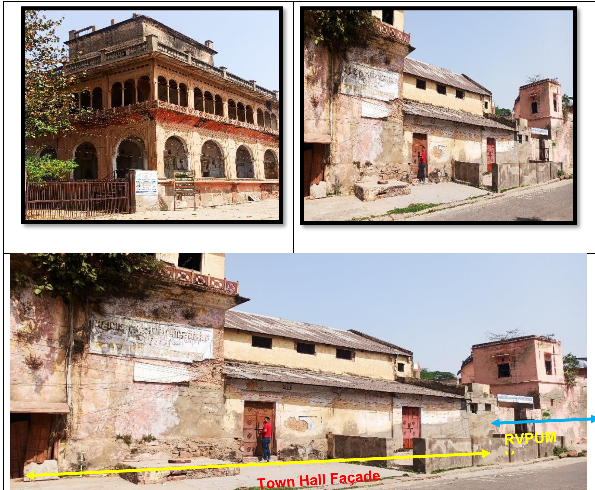
Figure 2: Present Condition of Town Hall and government school (RVPUM) overlooking the road
