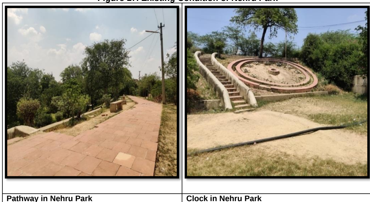
Figure 17. Existing Condition of Nehru Park
