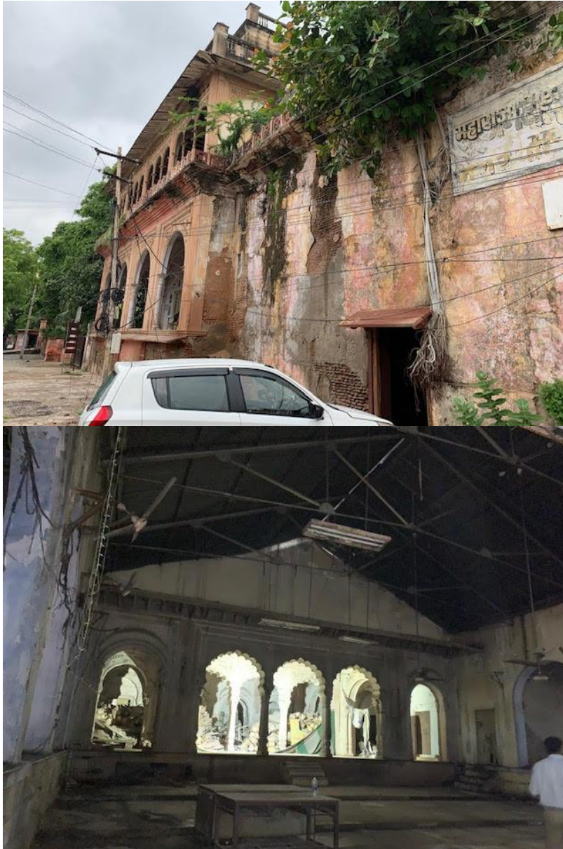
Phase I of the building is the two storied building with the arcade; Phase II of the building is a plain masonry structure which houses a large hall roofed with trusses and corrugated sheets.
