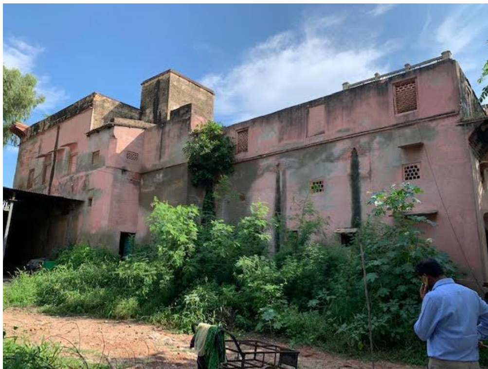
Existing Condition of Town Hall
