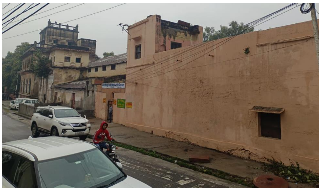
Existing Condition of Government RVPUMV School
