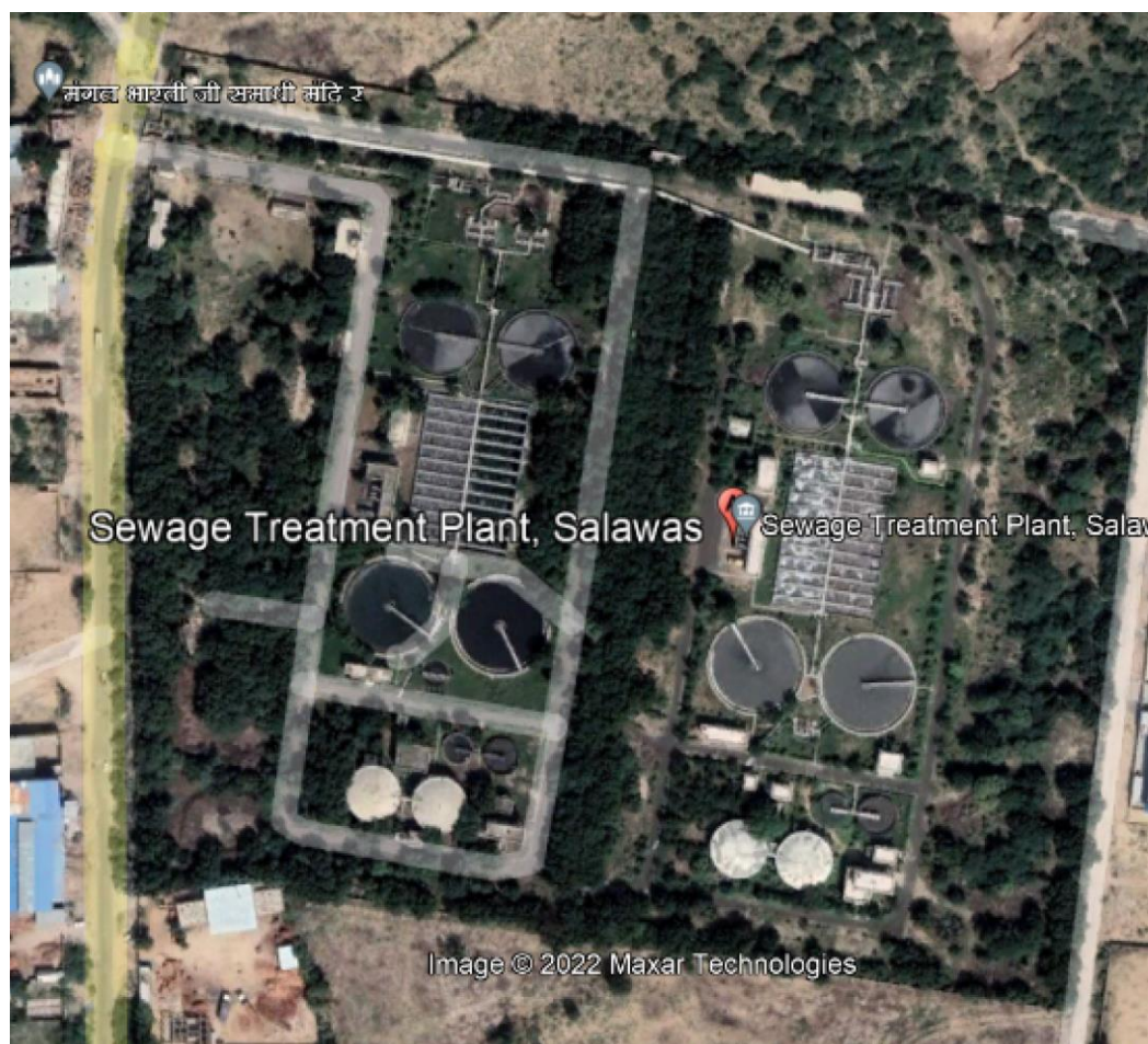
STP Salawas. Google Earth image dated - 10.11 2021
