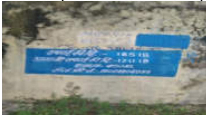
Figure 15 : RCC GLSR on hill near AEN office for new abadi zone
