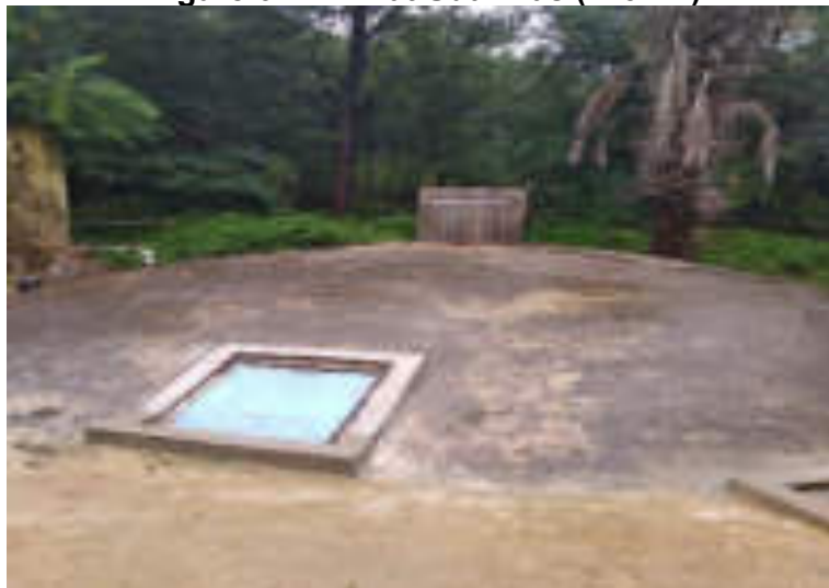
Figure 7 : CWR at Udaivilas (113 KL)
