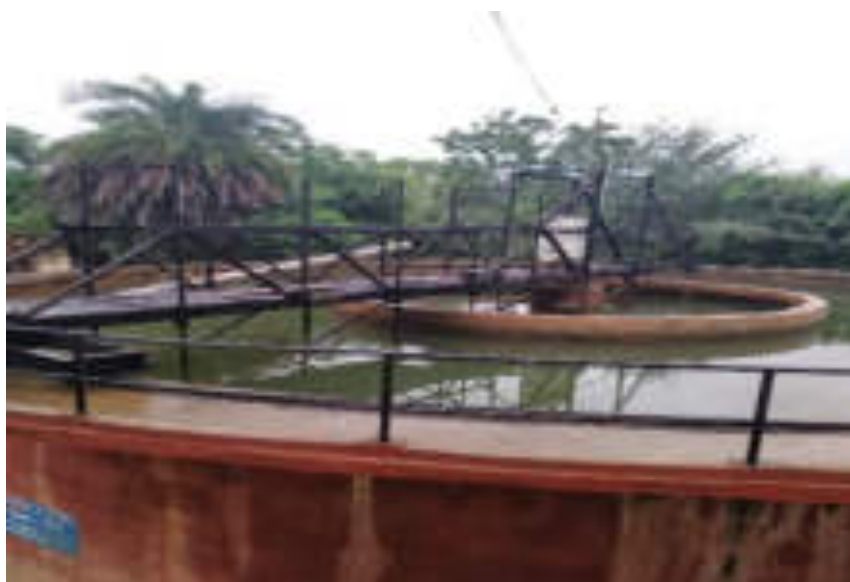
Figure 2 : Udai vilas clarifloculator
