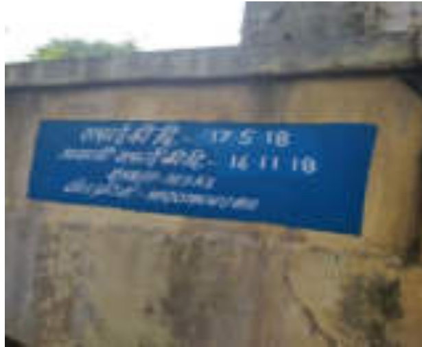
Figure 14 : Masonry GLSR on hill at AEN office for city zone
