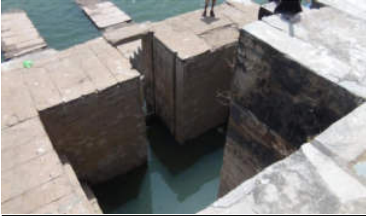
Fig. 11 Intake as Edward Sagar Dam
