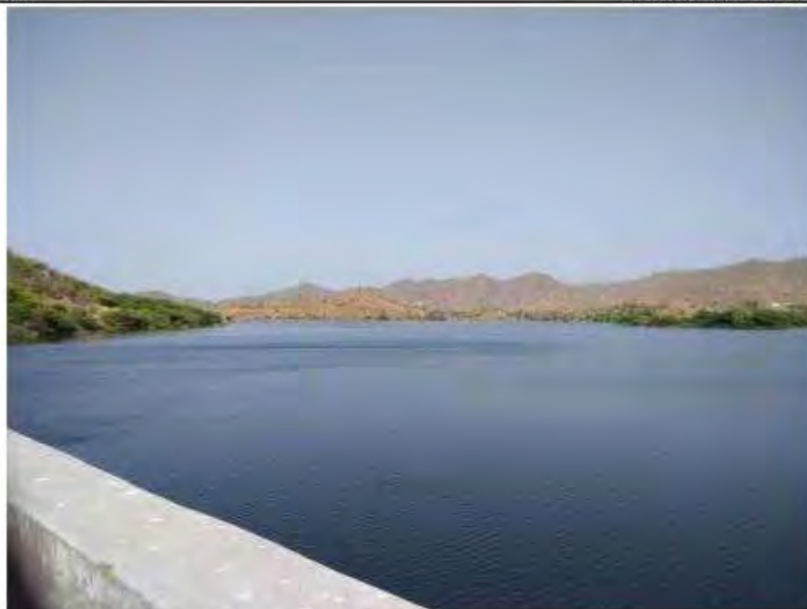
Photo 2 Bhaisa Singh Dam view Surrounded by Hills
