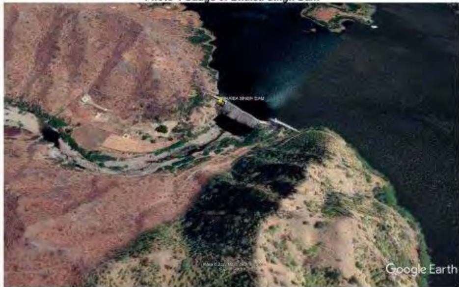
Photo 5 Google Image of Top view of Bhaisa Singh Dam Wall
