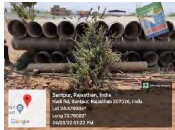
AC pipe encountered at STP Santpur site
