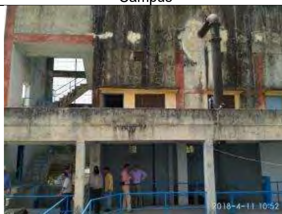
Existing building of WTP at AEN Campus
