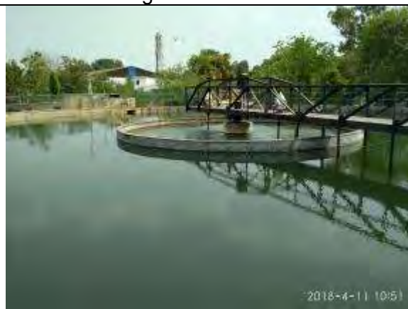
Clariflocculator at Existing WTP at AEN Campus
