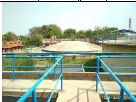
Existing WTP at AEN Campus
