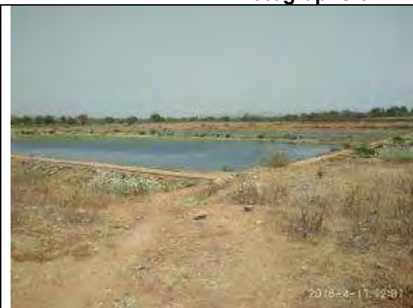
WSP at Existing STP
