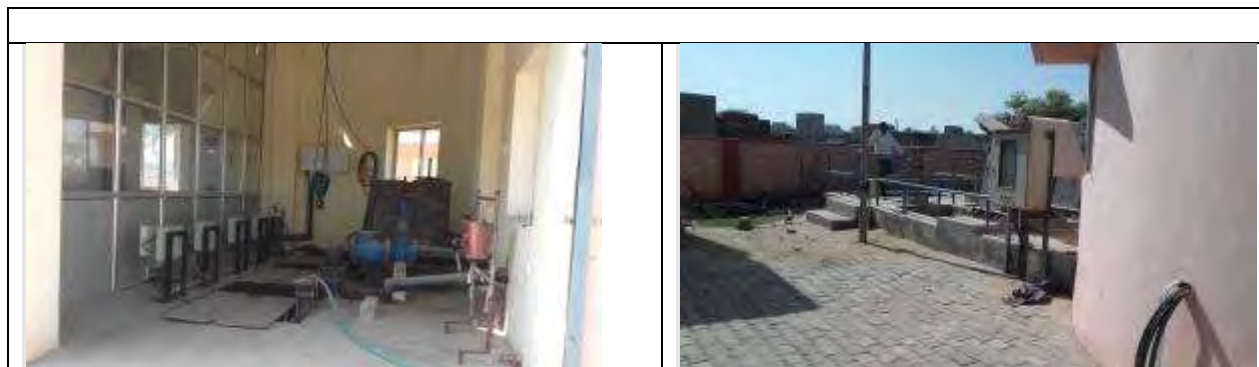
Existing SPS-2 (1.3 MLD) at Kharia Talab
