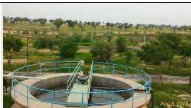
Existing STP at Mela Maidan
