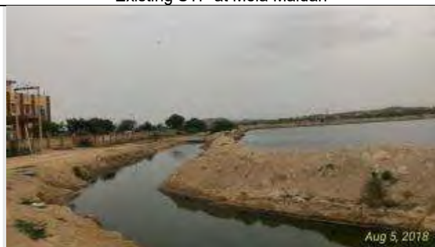
Effluent discharge of existing STP in lagoon
