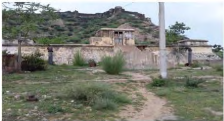
RCC GLSR on hill behind PWD Office
