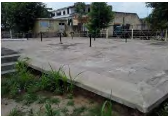
Masonry CWR near AEN Office
