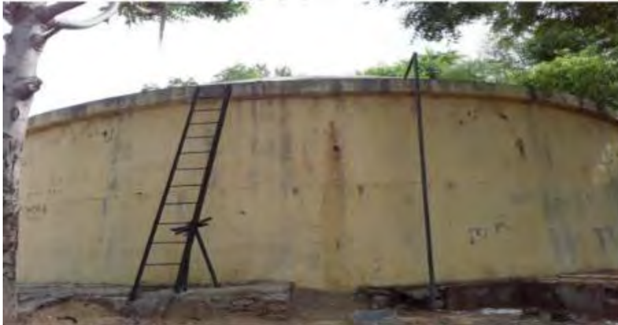
Masonry GLSR on hill behind PWD Office
