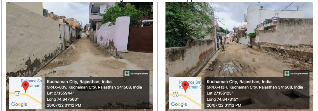
WS &amp; Sewerage laid at Padampura Road
