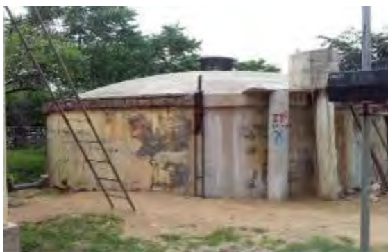
RCC CWR at Panchwa Road
