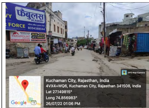
WS & Sewerage laid at Chungi Didwana Bus Stand Road
