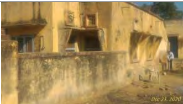
Existing old building proposed for demolition for construction of CRMC at PHED Aen campus
