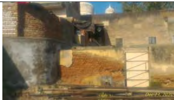
Habitations beside the proposed CRMC site
