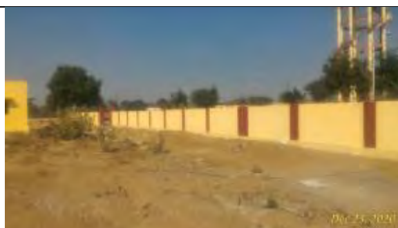
Site is having boundary wall
