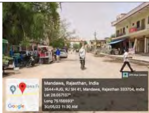
Trenchless Sewer Work from Dhigal Mod to PHED J.En. campus SPS on Fatehpur Bypass-Completed
