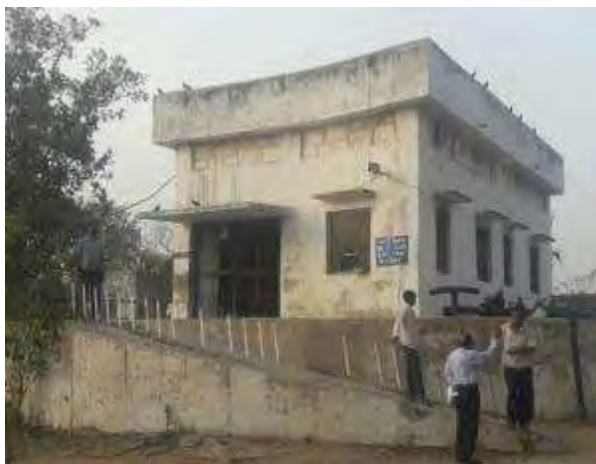
ANGOR HEAD WORKS ANGORE DAM
