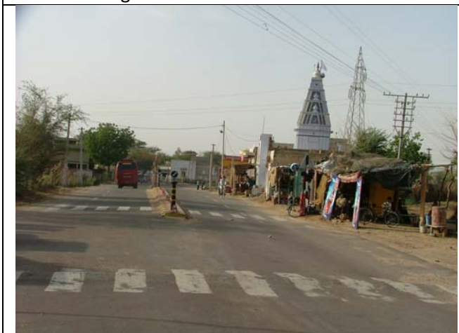
Approach Roads to Railway Crossing
