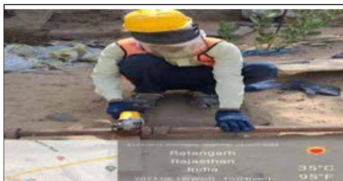
Good Practice: Safety during Bar cutting works
