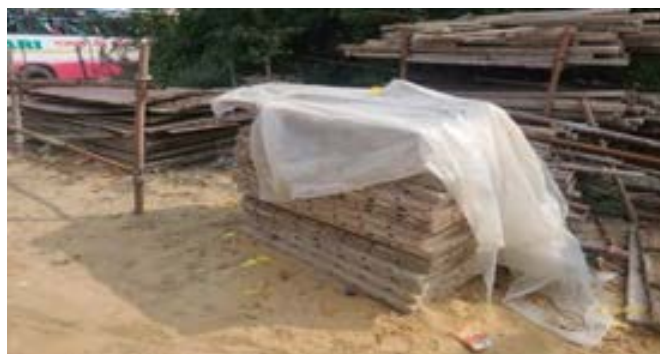
Good Practise: Material Stacking at Site
