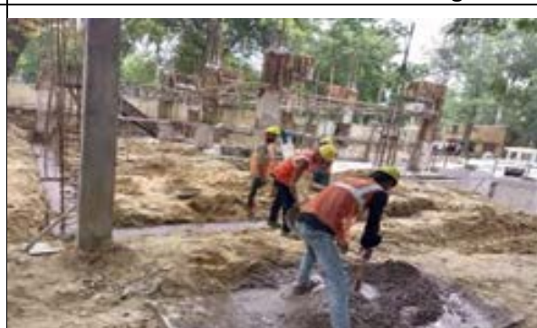
Good Practise workers working with PPEs
