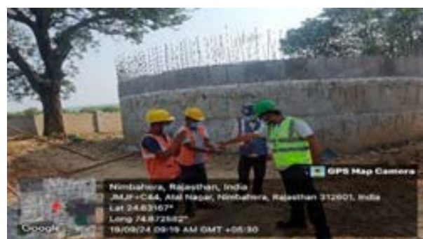
Hand Sanitization activity of workers at site Nimbahera
