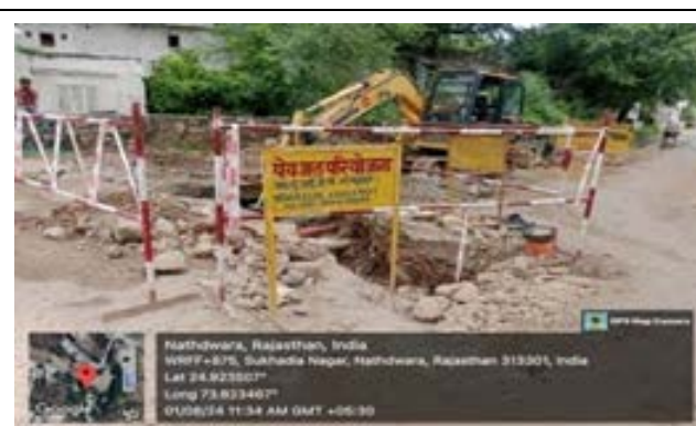
Good Practise: Hard Barricading at work site
