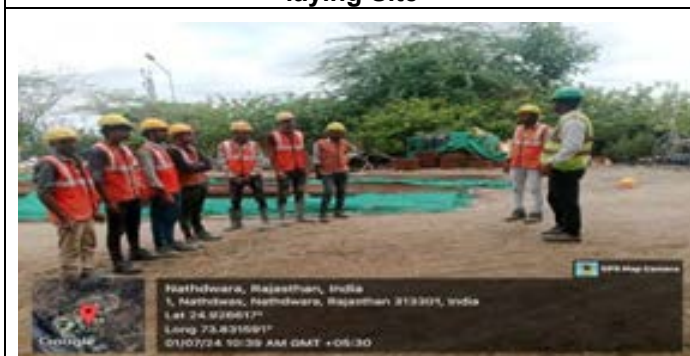
Good Practise: workers working with PPEs at site
