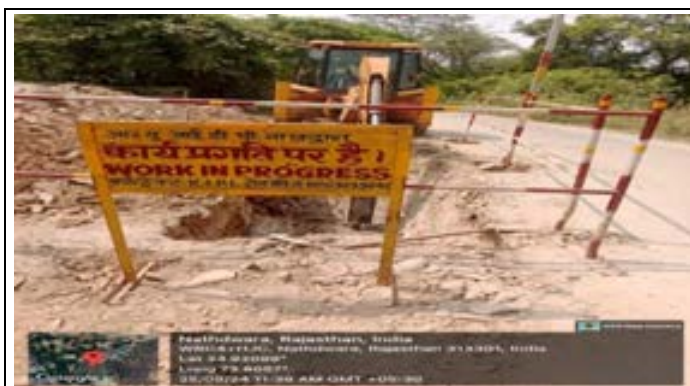
Good Practise: Barricading & sign board at Pipe laying Site
