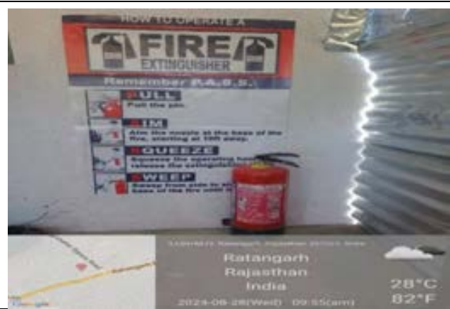
Good Practise:Availibility of Fire Extinguisher at site
