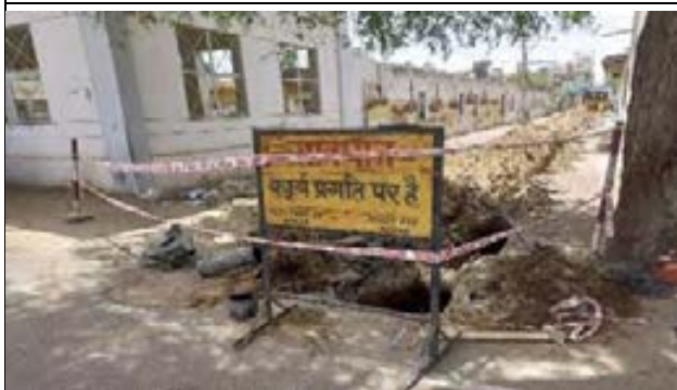
Good Practise: Barricading at work site
