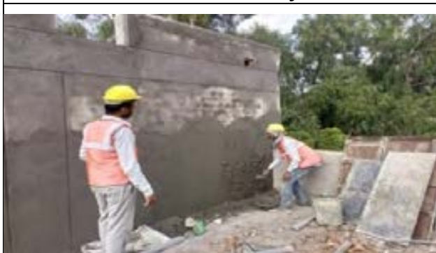
Good Practise: House Keeping at work site
