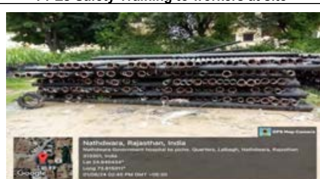
Good Practice: Material Stacking at site
