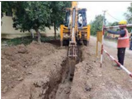
A view of water supply excavation & pipe laying work under progress
