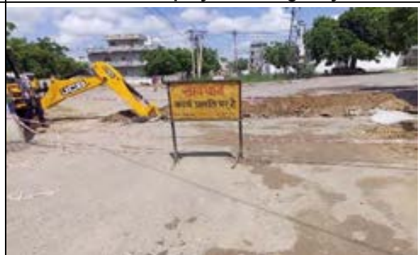
Good Practise: Excavation &amp; trenching at site
