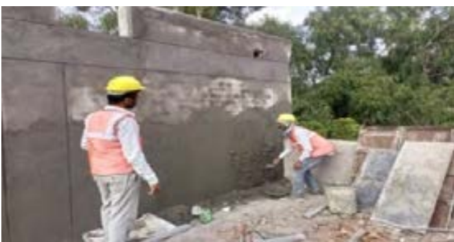
Good Practise House Keeping at work site
