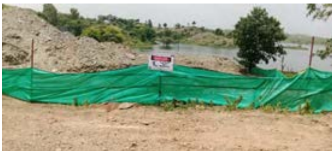
Good Practise: Hard Barricade with Sign Board
