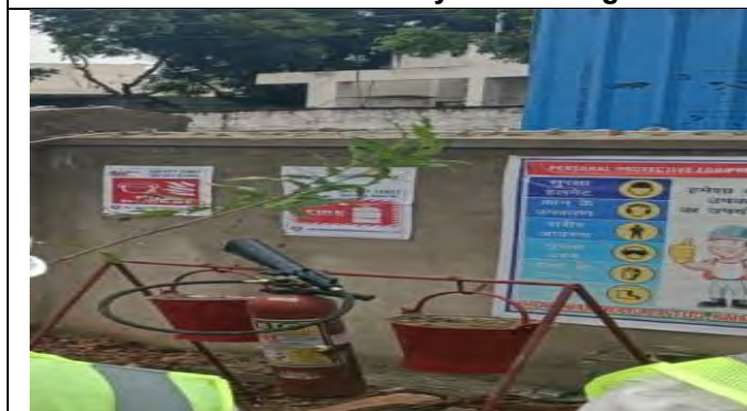
Good Practice: Fire extinguisher & Bucket at site
