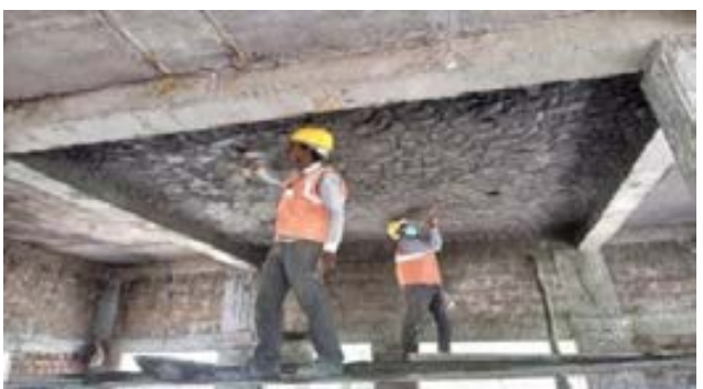
Good Practise workers working with PPEs
