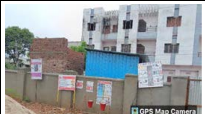
Good Practice: Display of Safety Sign Board
