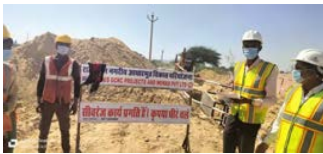
Good Practice Barricading
