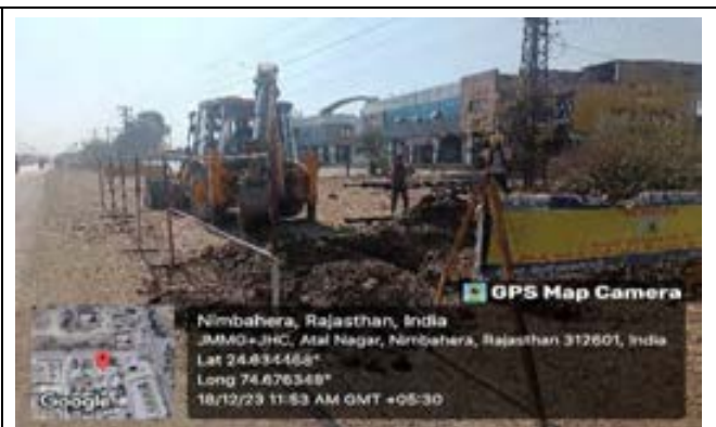
Good Practice: Excavation & Trenching
