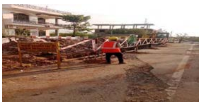
Good Practice: Use of flag during Road Diversion at Pipe laying site
