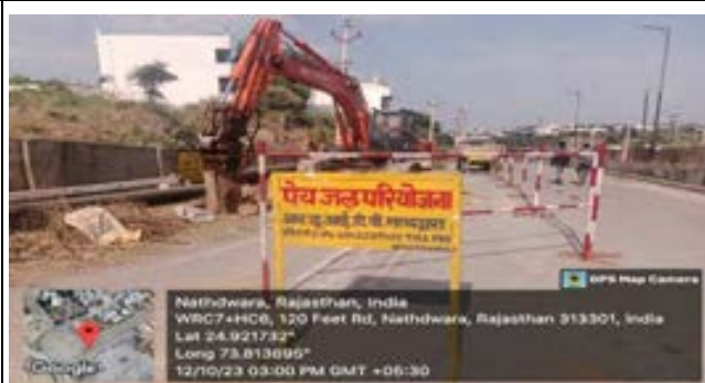
Good Practise: Hard Barricading at work site
