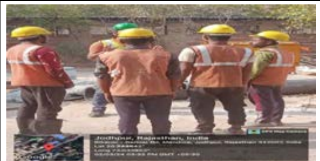
Training on Work at Height safety
