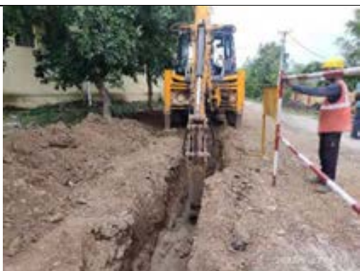
A view of water supply excavation &amp; pipe laying work under progress
