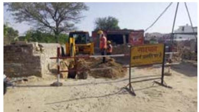
Good Practise Excavation &amp; trenching at site
