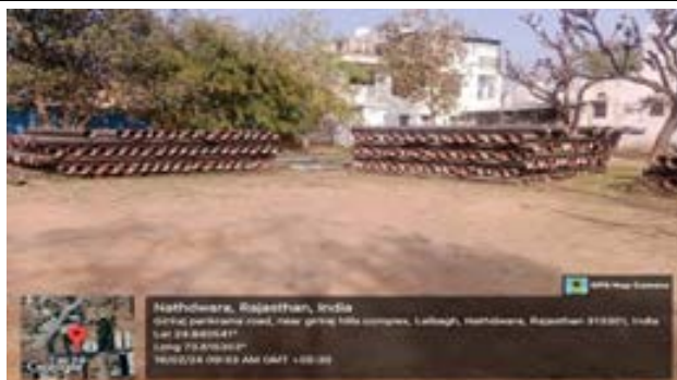
Good Practice: Material Stacking at site
