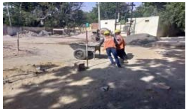
Good Practise Material handling
