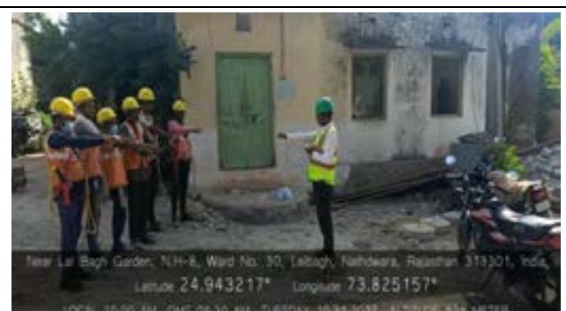
Safety Pledge to workers at site
