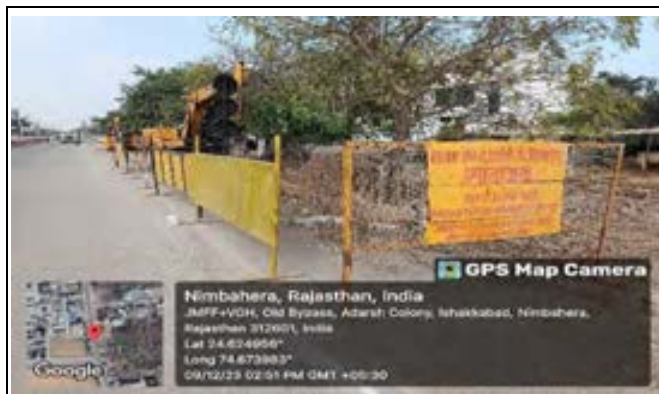
Good Practice: Barricading
