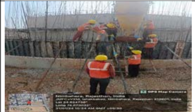
Good Practice: Workers working with PPEs
