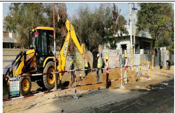
Good Practice Excavation & trenching
