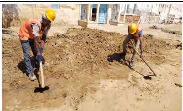
Good Practice House Keeping
