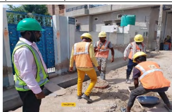
Good Practice House Keeping
