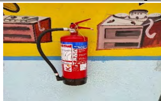
Good Practise - Posters &amp; Sign Board &amp; Fire extinguisher
