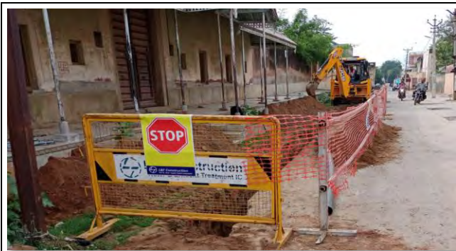
Good Practice Barricading
