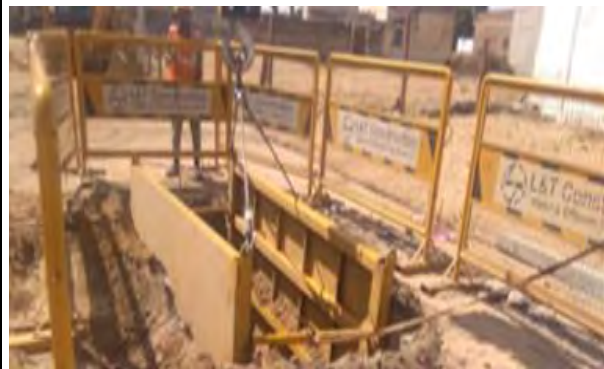
Good Practice Excavation & trenching
