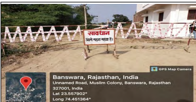
Good Practice Barricading
