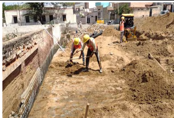
Good Practice House Keeping
