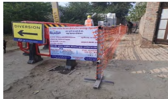
Good Practice Excavation &amp; trenching
