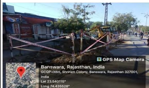
Good Practice Excavation & trenching
