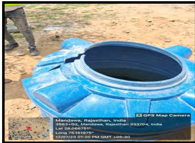
Water tank was found in damage condition
