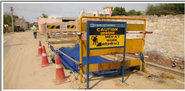
Good Practice Barricading
