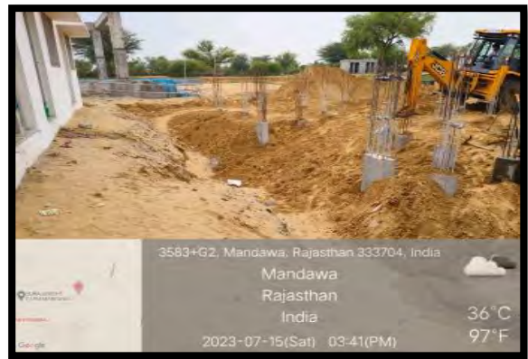
Low laying structural area filled up with excavated earthwork to prevent uneven surface area.
