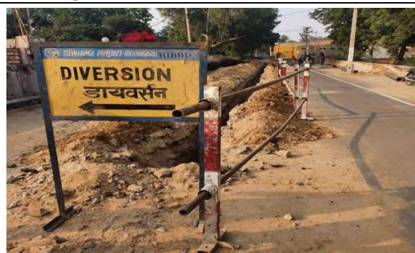
Good Practice Excavation & trenching
