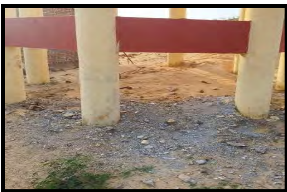
All sharp edges loose tin material covered and placed with proper weight load to prevent injury. Unwanted debris removed from work site.
