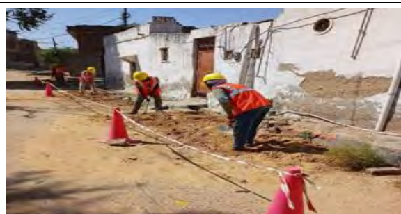
Good Practice House Keeping
