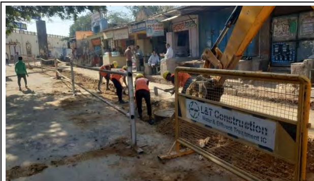
Good Practice Barricading
