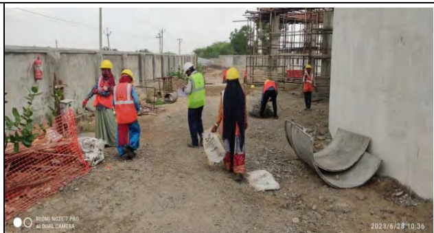
Good Practice House Keeping
