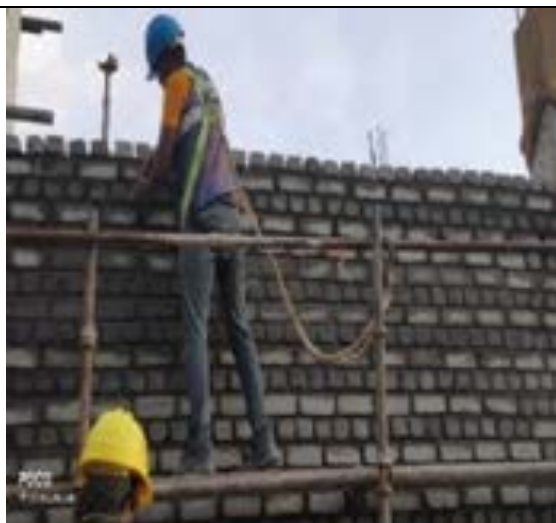
Action taken: PPEs provided to everyone and Labours following proper safety protocols while working on the site.
