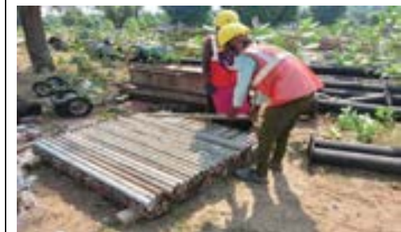
Good Practise: Material handling
