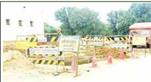
Good Practise Excavation & trenching
