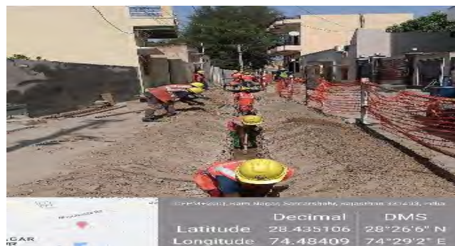
Good Practise Excavation &amp; trenching
