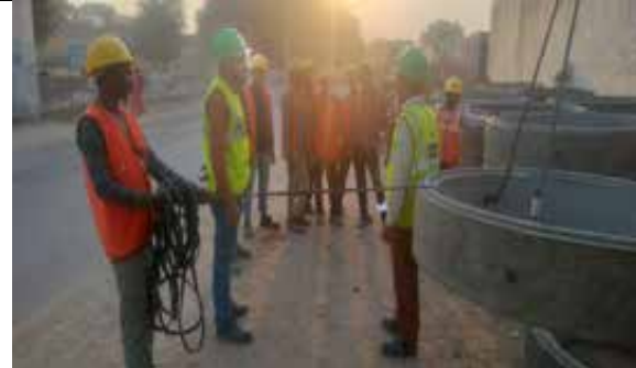
Good Practise Material handling
