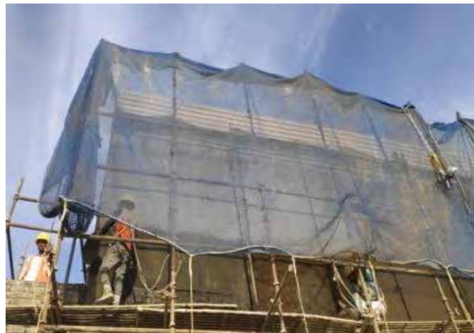
Good Practice; Required PPE's and secondary Protection has been Provided
