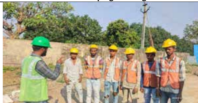
Training On Material Handling
