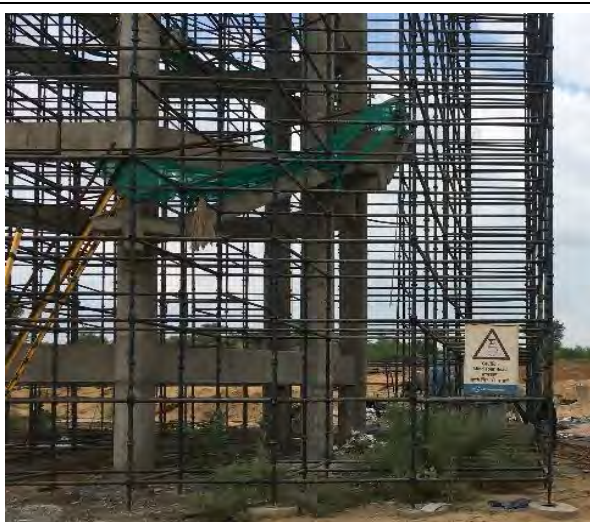
Good arrangement of scaffold at TESR at 2.3 MLD STP site, Sardar Shahar
