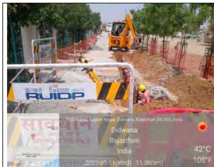
Good Practise Barricading
