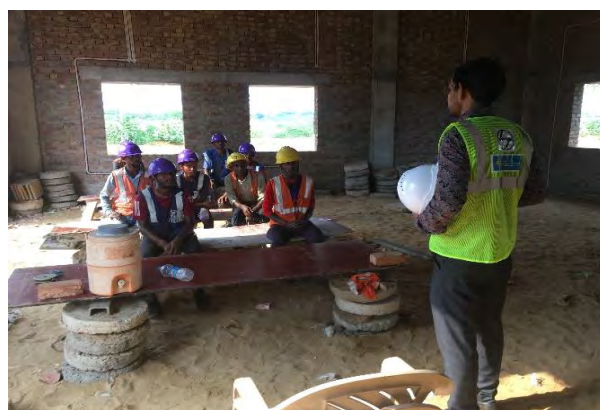
Safeguard Orientation of workers at 3.4 MLD STP construction Site (Sardar Shahar)
