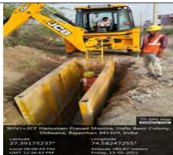
Good Practise Excavation &amp; trenching
