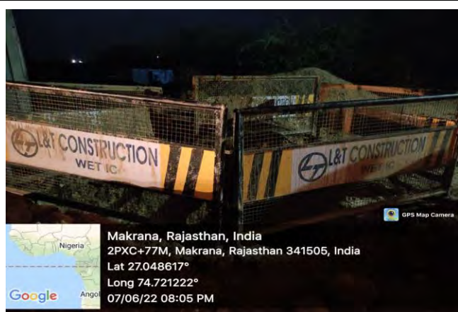
Good Practise Barricading
