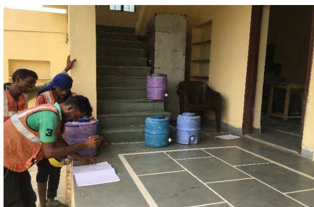
Safeguard Orientation at Working Site "Sewer Pipe Laying Site-Zone: 2-Bahadur Colony (Sardar Shahar)
