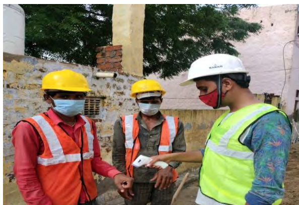
Thermal Screening of workers at site (Mandawa)
