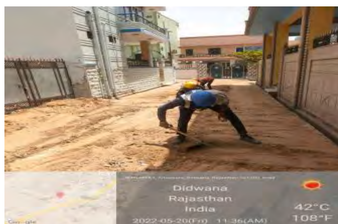
Good Practise House Keeping
