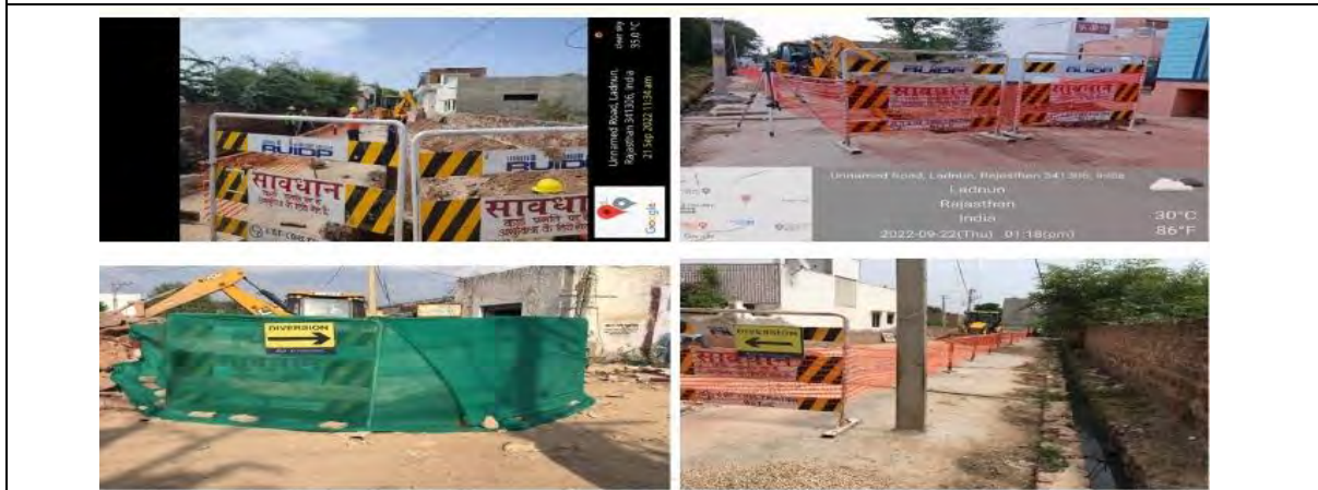
Good Practise – Hard Barricading with Signage Board
