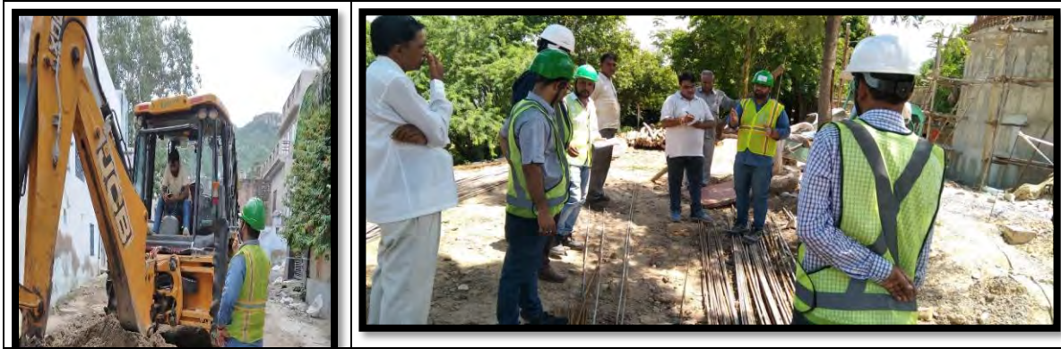
Abu Road Town (Site Visited on dated 18.08.2022)
