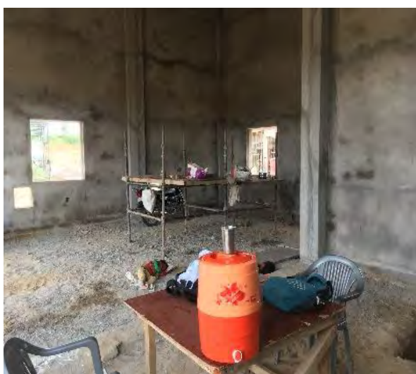
First Aid Room with one bed was observed at STP site at 3.4 MLD STP Site
