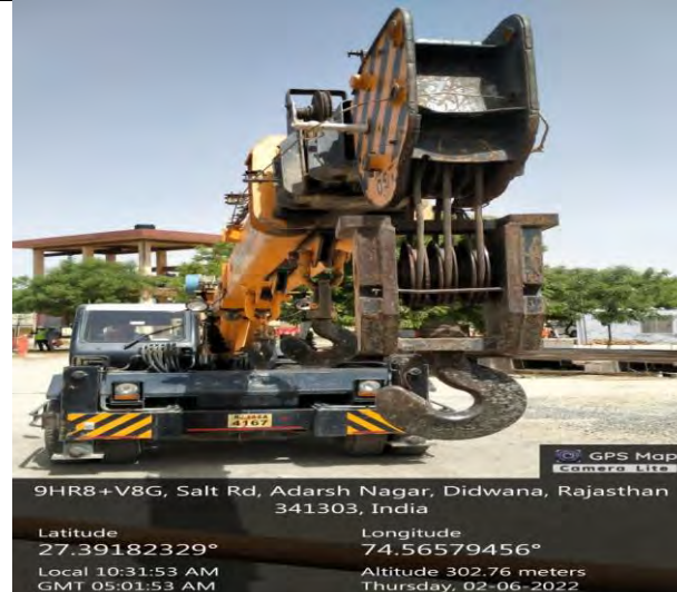
Good Practise Material handling
