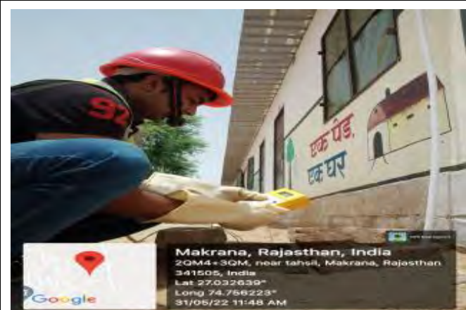
Good Practise Earth Resistance testing
