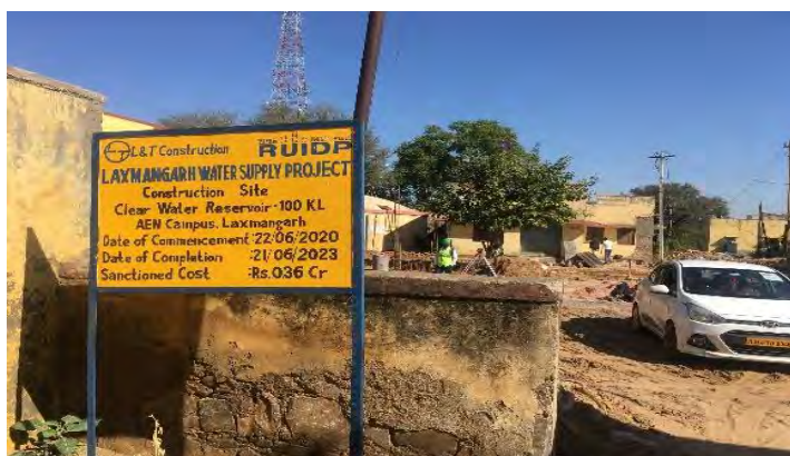
Project Information board at CRMC Site, Laxmangarh;
