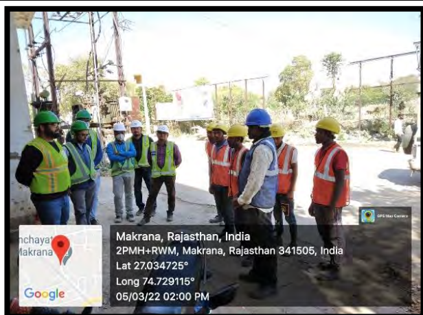
Safety Training at working site for Site Staff and Labours (Work at Height)
