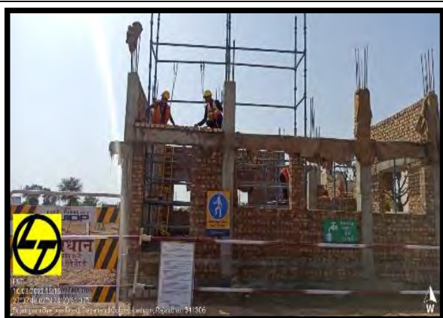
Work at height safety @ CWR; Ladnu
