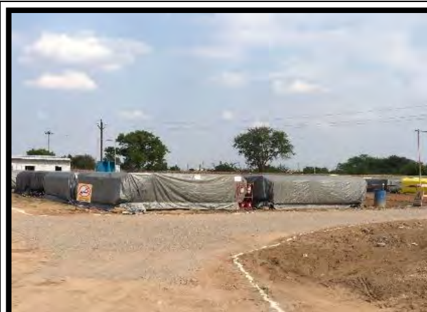
Proper Material Stacking @ Stock Yard; Ladnu
