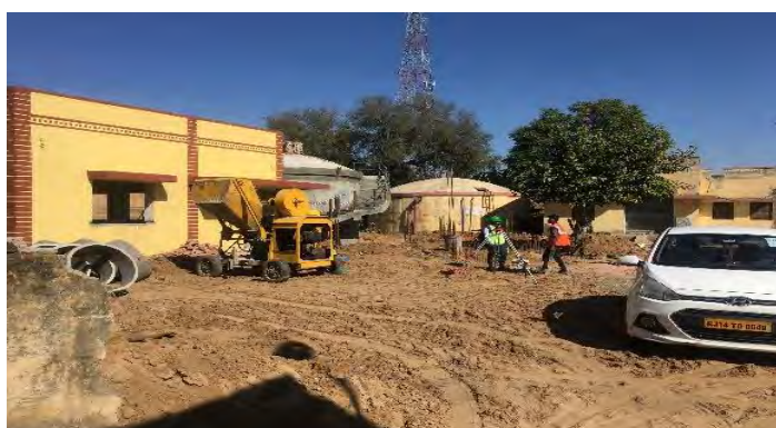
Proper site clearance at CRMC Building, Laxmangarh
