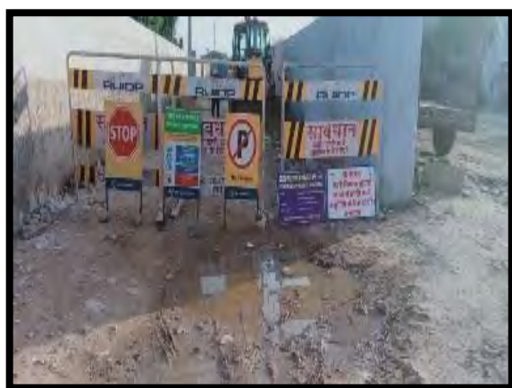
Site Specific Safety Signage board was noticed at site with emergency contact details and toll-free number
