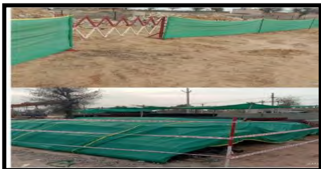
Proper Material stacking of DWC & HDPE Pipe for water line connection @ Stock yard
