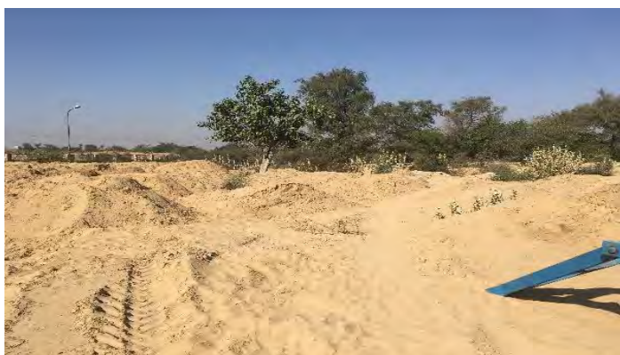
Excavated soil storage near the CWR site in PHED Campus on Hanumangarh Road.
