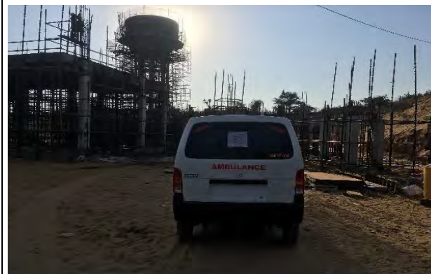
Ambulance at 3.8 MLD STP Site on Old NH-11
