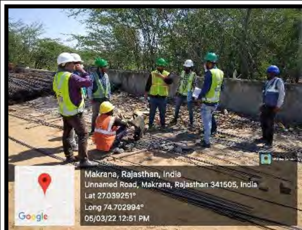
Safety Training at working site for Site Staff and Labours (Inspection and Use of Electrical Tools)
