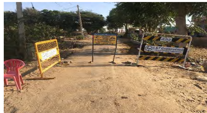
Barricading for diversion of road traffic at truck line laying
