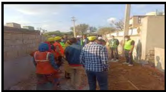
Safety Training of Contractor Site Staff at Labour water line connection area on Manual Handling Material at site.
