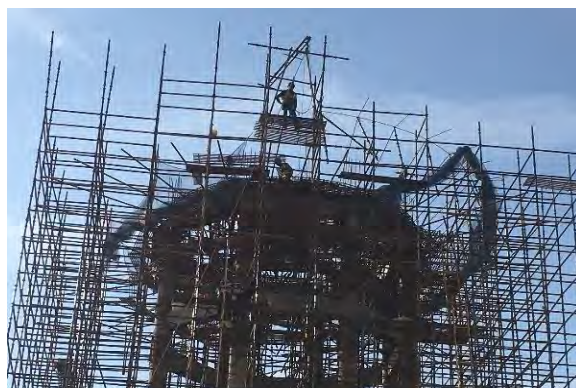
Safety belt and other PPEs at working on height of TEER, 3.4 MLD STP in North Campus of Gaushala
