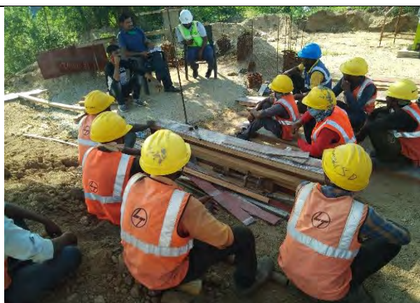
Photographs of Training Orientation at 1.7 MLD STP Woking Site on Revdar Road, Sirohi 05.10.2021
