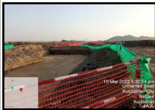
Proper hard barrication of excavated structural area
