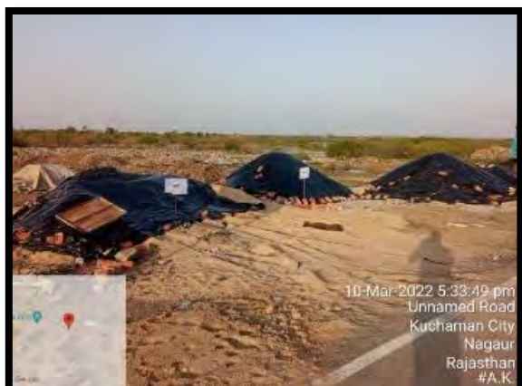
Proper material tarpaulin coverage of aggregate at site
