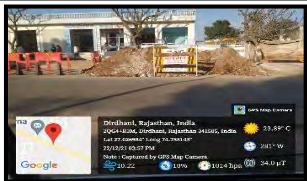
Sewerage Line work safely with Cautionary Board
