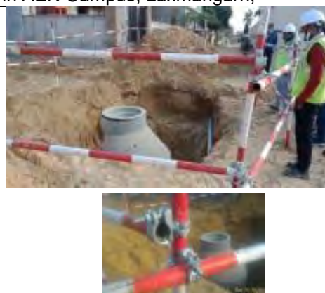
Proper Pipe barricades with steel fixtures/clamps, Laxmangarh
