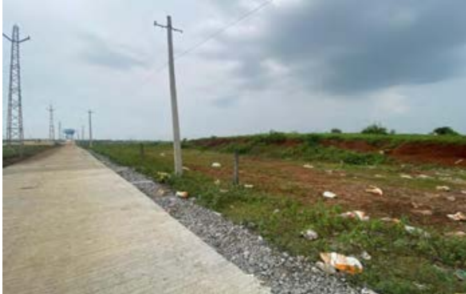
Paved CC Road from Gupt Ganga Mandir Marg to STP
