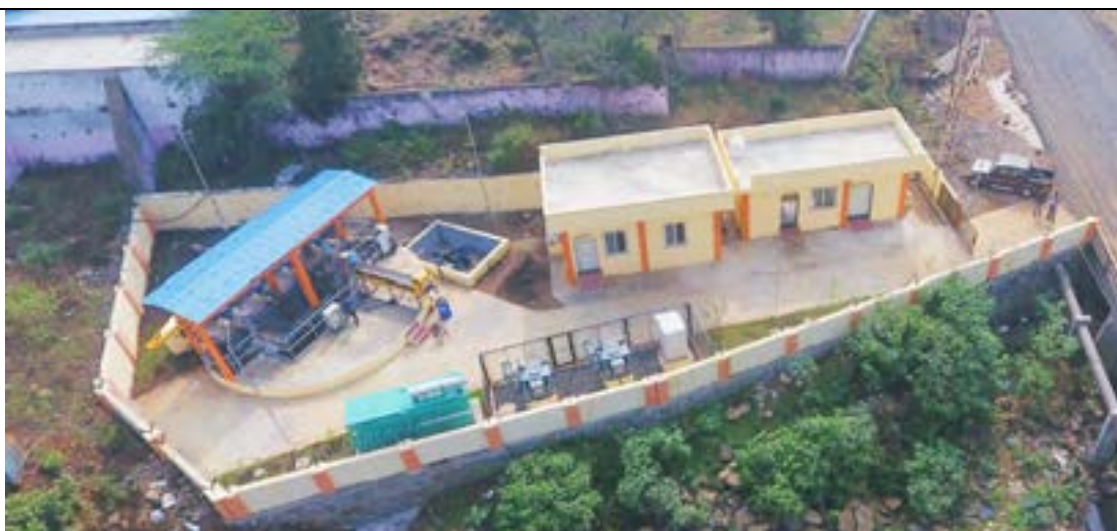
SPS-7 MLD on Qila Road-Pratapgarh
