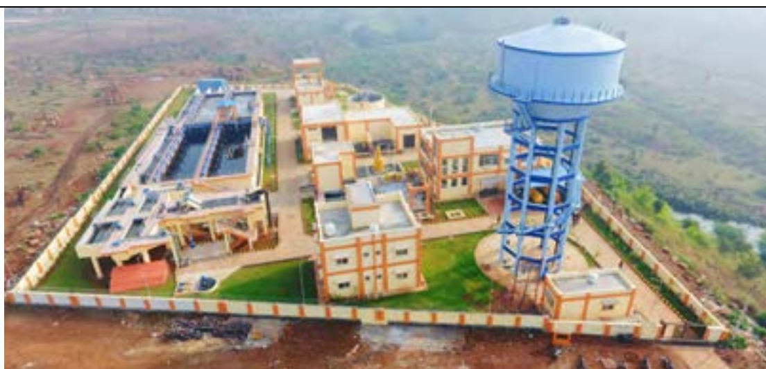
STP-7 MLD near new by-pass Gupt Ganga Road, Pratapgarh
