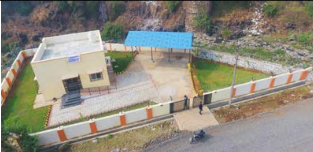
CRMC-2, near SPS (7 MLD) on Qila Road-Pratapgarh
