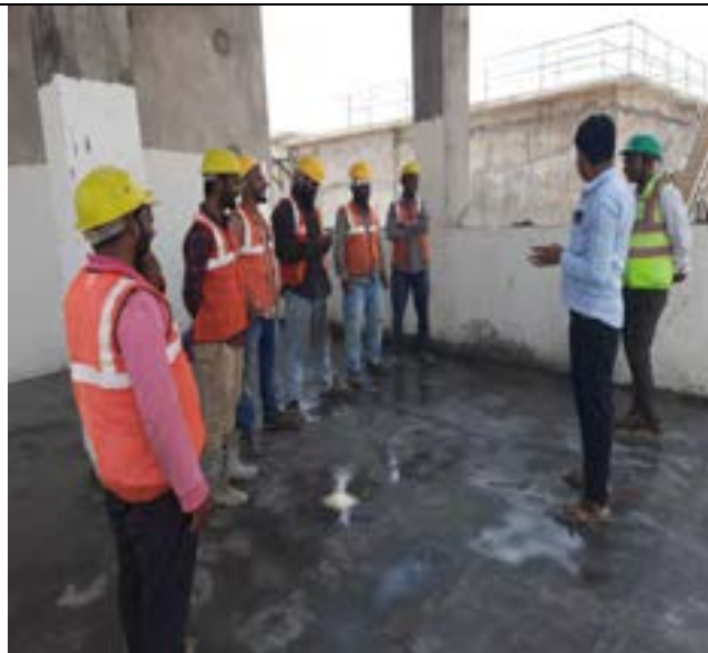
Discussing health and safety with project labour. Date 11-04-2023
