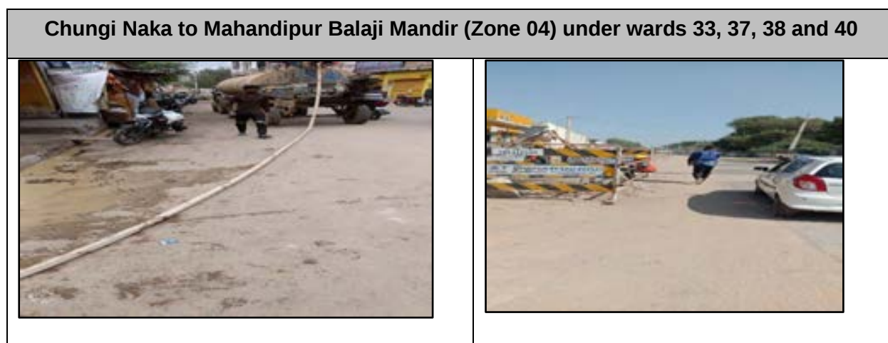
Figure 13: Site Photographs of Additional length (2.92 km) covered under Trenchless (HDD Method)
