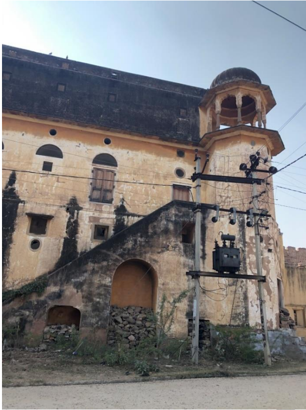
Source 29 Author Figure 51 showing rear elevation of building (Amar Mahal) adjacent to Khetri Trust
