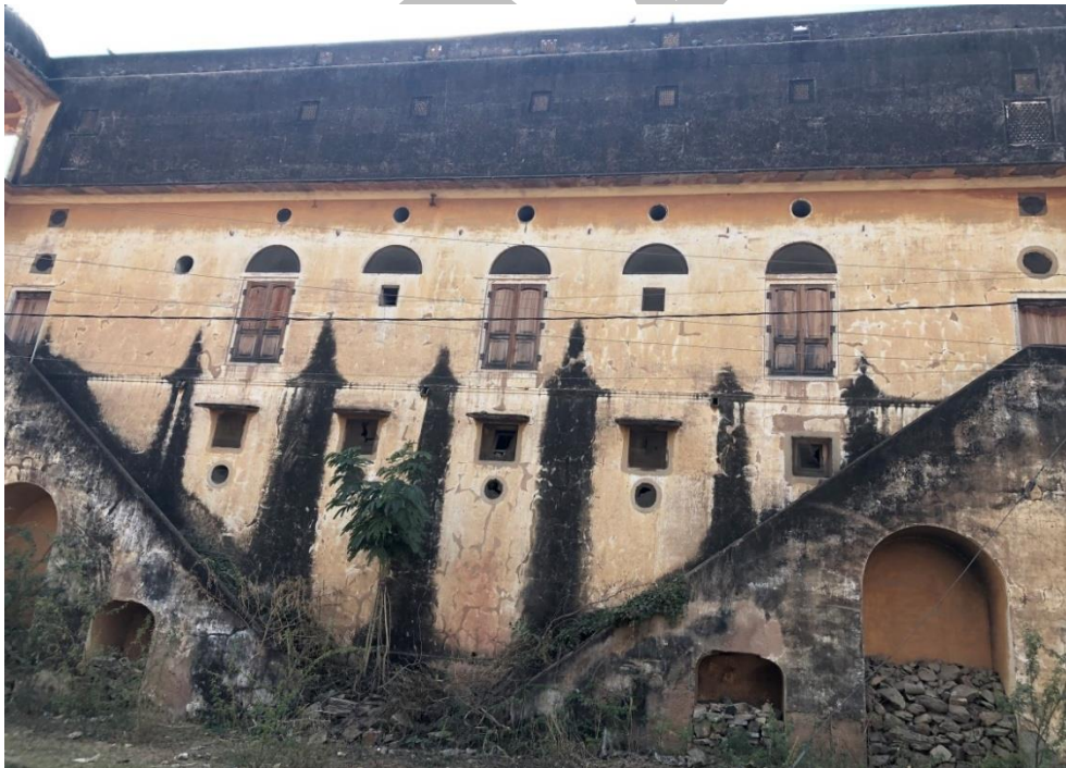
Source 28 Author Figure 50 showing rear elevation of building (Amar Mahal) adjacent to Khetri Trust
