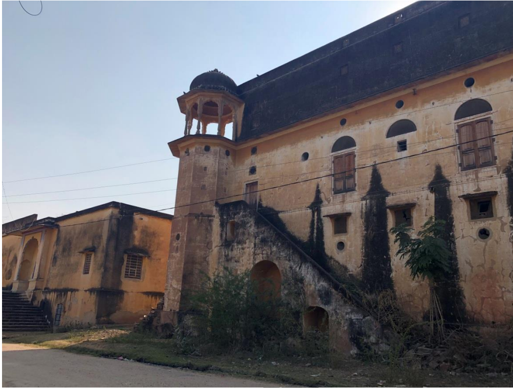
Source 27 Author Figure 49 showing rear elevation of building (Amar Mahal) adjacent to Khetri Trust
