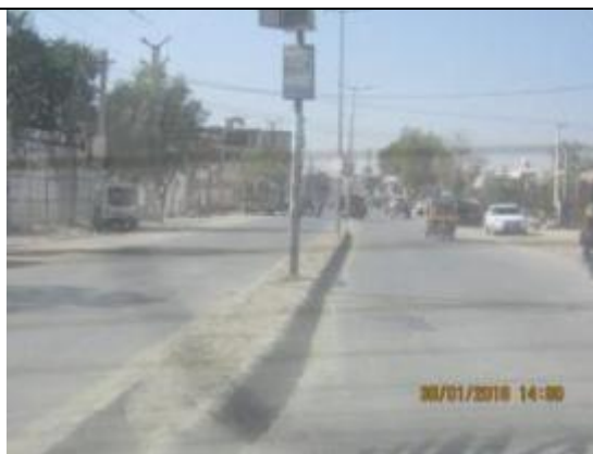
Main city road in Makrana
