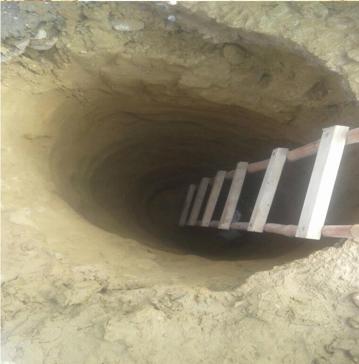
Maintenance work carried out for uPVC line leakage repair at Ward-05, Pipe Line located at an depth of more than 12ft. Ladder being used for access of repair work.
