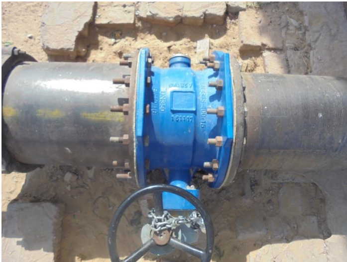
Existing Transmission main Pipe Line in workable condition.
