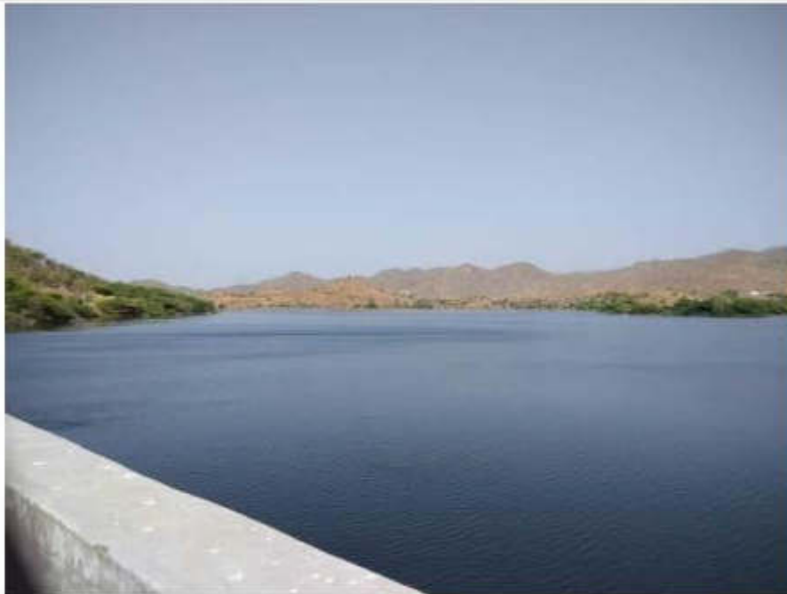
Photo 2 Bhaisa Singh Dam view Surrounded by Hills
