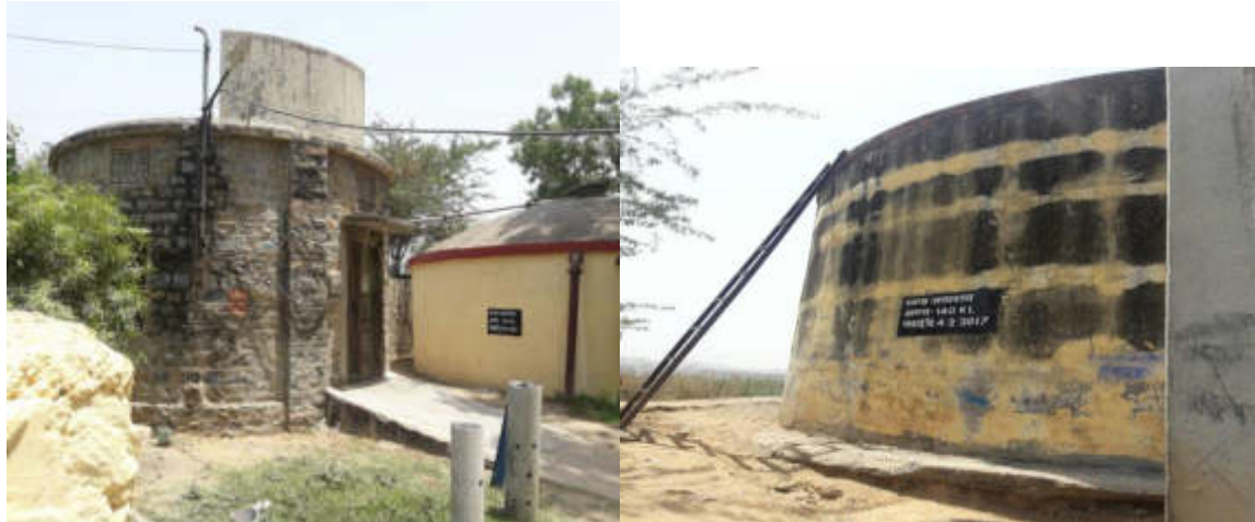
MARKET AREA PUMP HOUSEMANPURA GLSR
