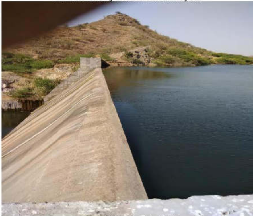
Photo 3 Bhaisa Singh Dam Wall
