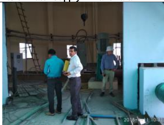
Existing Intake at Mahi Dam
