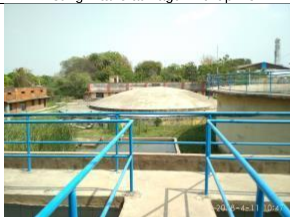
Existing WTP at AEN Campus
