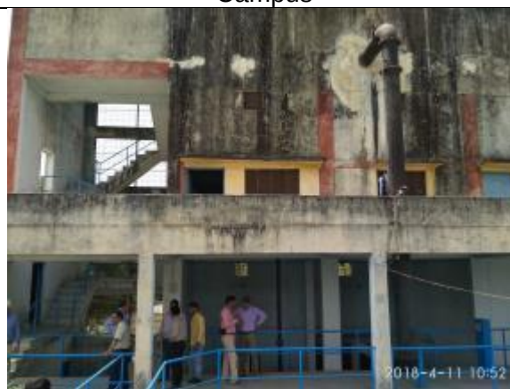
Existing building of WTP at AEN Campus
