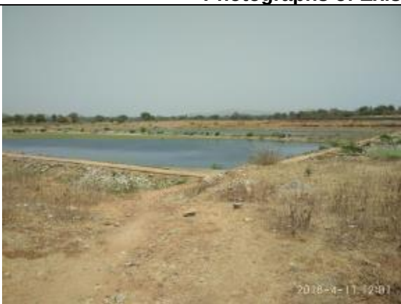
WSP at Existing STP
