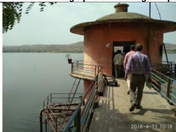
Existing Intake at Kagdi Pickup weir
