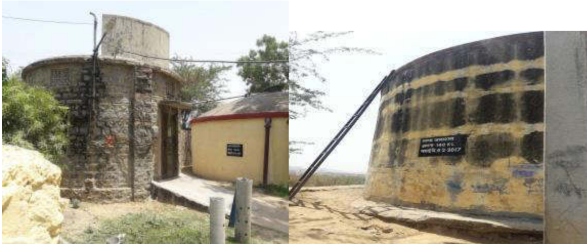
MARKET AREA PUMP HOUSE MANPURA GLSR
