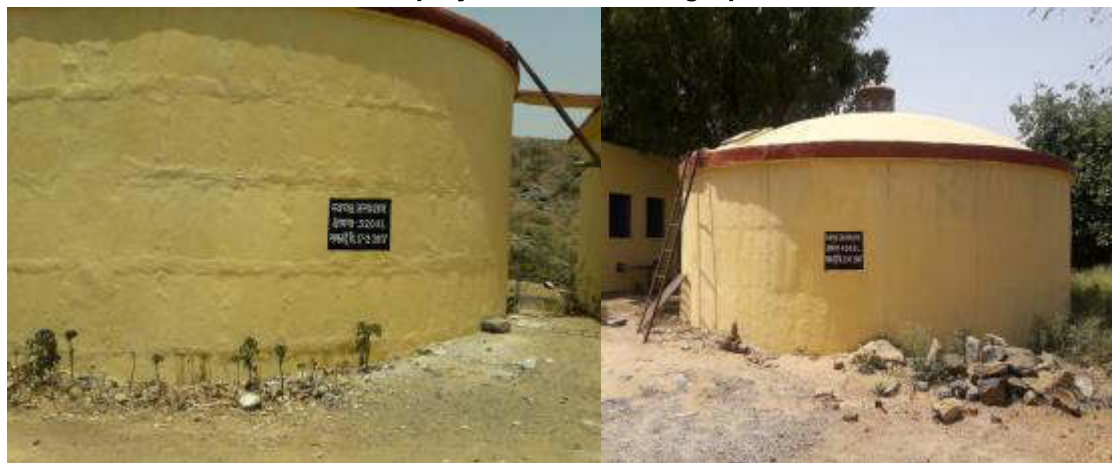
GANDHI NAGAR PUMP HOUSE
