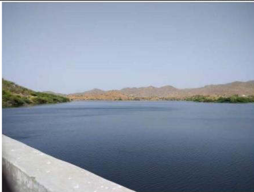
Photo 2 Bhaisa Singh Dam view Surrounded by Hills
