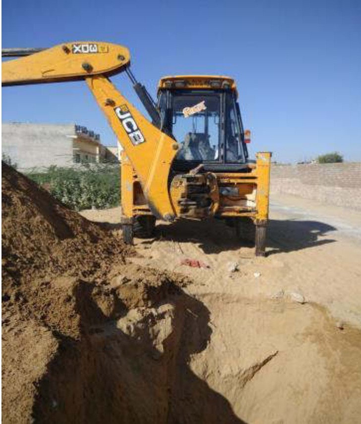
JCB being used for excavation work at Ward No 12 for Distribution Network
