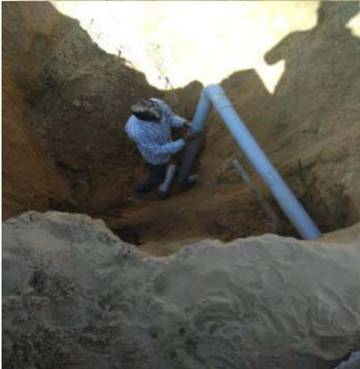
Existing Distribution Line connection work at Ward No 14.
