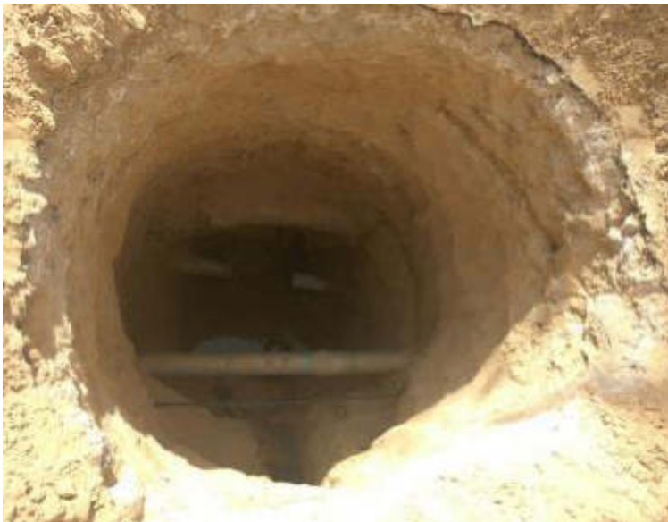
Maintenance work carried out for uPVC line leakage repair at Ward-23, Pipe Line located at an approx depth of 7-8ft
