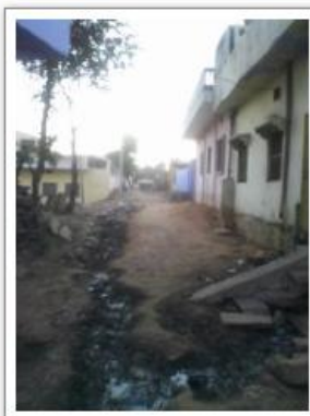
Proposed alignment pipe laying towards sps-4.jpg
